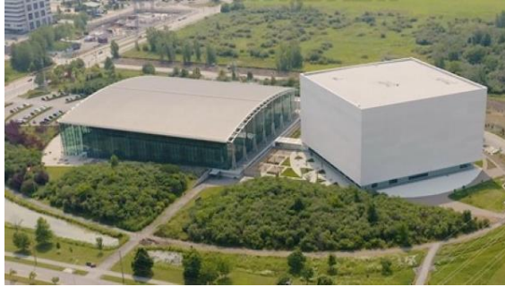
The Library and Archives Canada Preservation Centre and Preservation Storage Facility located at 635 du Carrefour Blvd., Gatineau, Québec.
