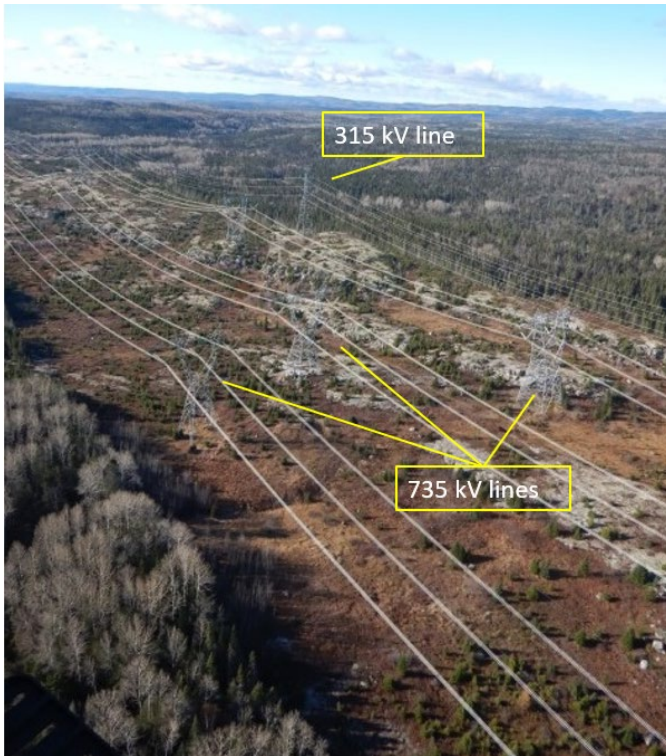
Figure 10. Aerial photo of the work area, near Les Escoumins (Source: TSB)
