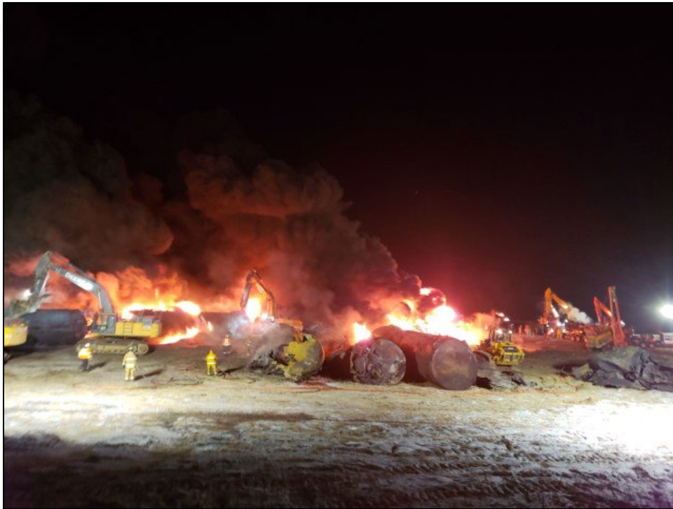
Figure 4. View of derailment site 18 hours after the accident (Source: TSB)
