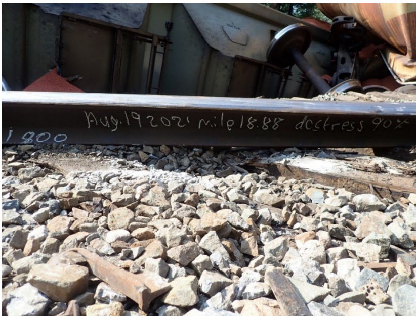
Figure 4. Chalk mark on the south rail indicating that work had recently been performed on the track (Source: TSB)
