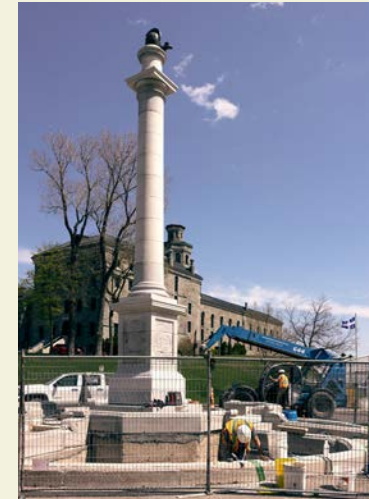
Restoration work of the Wolfe Monument
