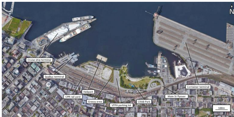
Figure 1: Pre-encampment Google Earth Pro satellite image of the vicinity of the encampment in VFPA v Brett . 3 Imagery © 2022 CNES / Airbus, Maxar Technologies, Map data © 2022. Used in accordance with Google Geo Guidelines. https://about.google/brand-resource-center/products-and-services/geo-guidelines/ .
