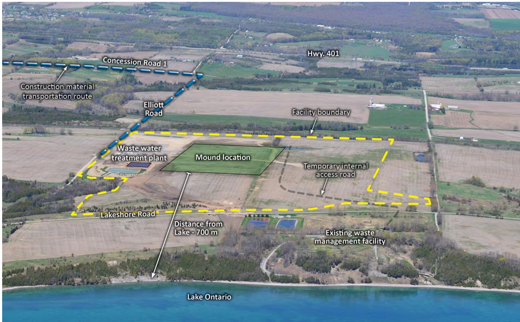
Figure 1.3: Aerial view of the Port Granby long-term waste management facility [22]
