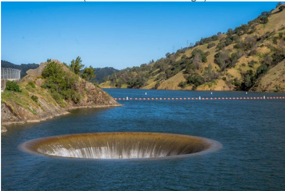
(c) Shaft spillway of the Monticello dam, USA (iStock.com/fusaromike)
