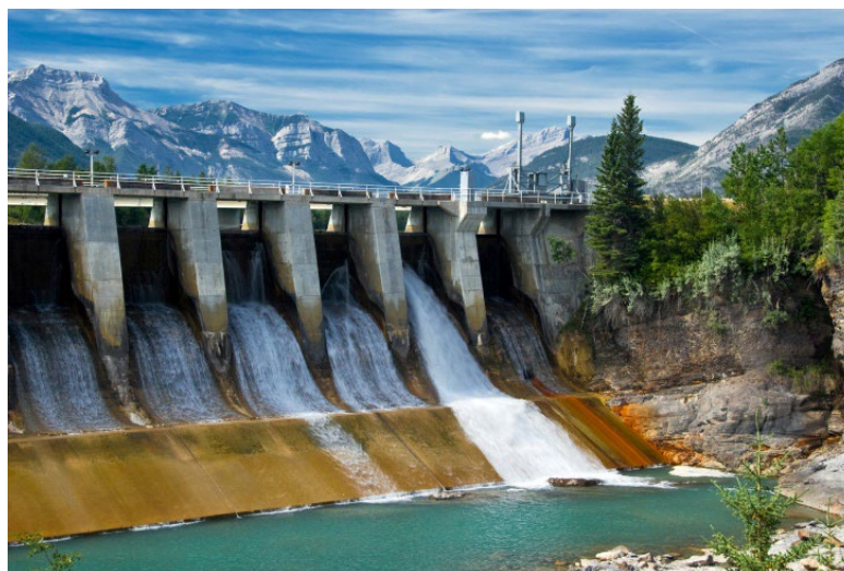
Figure 2.6 Water rushing through gates at the Kananaskis Dam in Alberta (iStock.com/Androsov)
