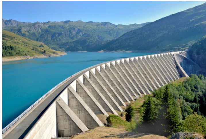
(b) Roselend Dam – a buttress dam in France (iStock.com/sanddebeautheil)
