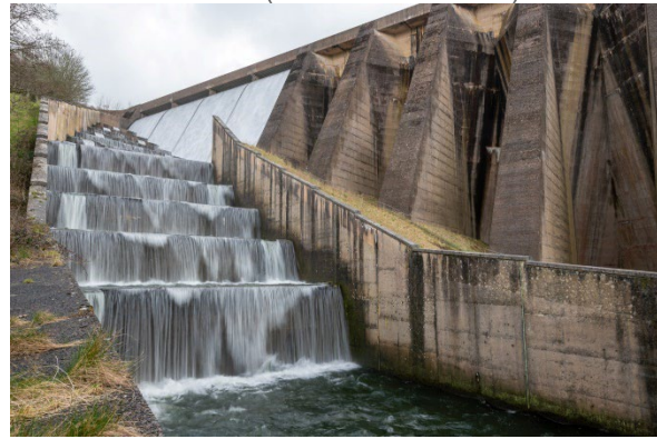
(d) Stepped spillway of the Wimbleball dam in Somerset, UK (iStock.com/Tom Meaker)
