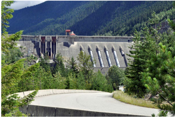
(a) Penstocks of the Canyon Dam in Revelstoke, B.C. (iStock.com/SeanFerguson)
