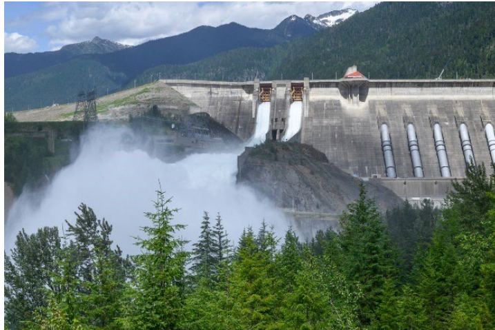
(a) Revelstoke Dam – a gravity dam in B.C. (iStock.com/James_Gabbert)
