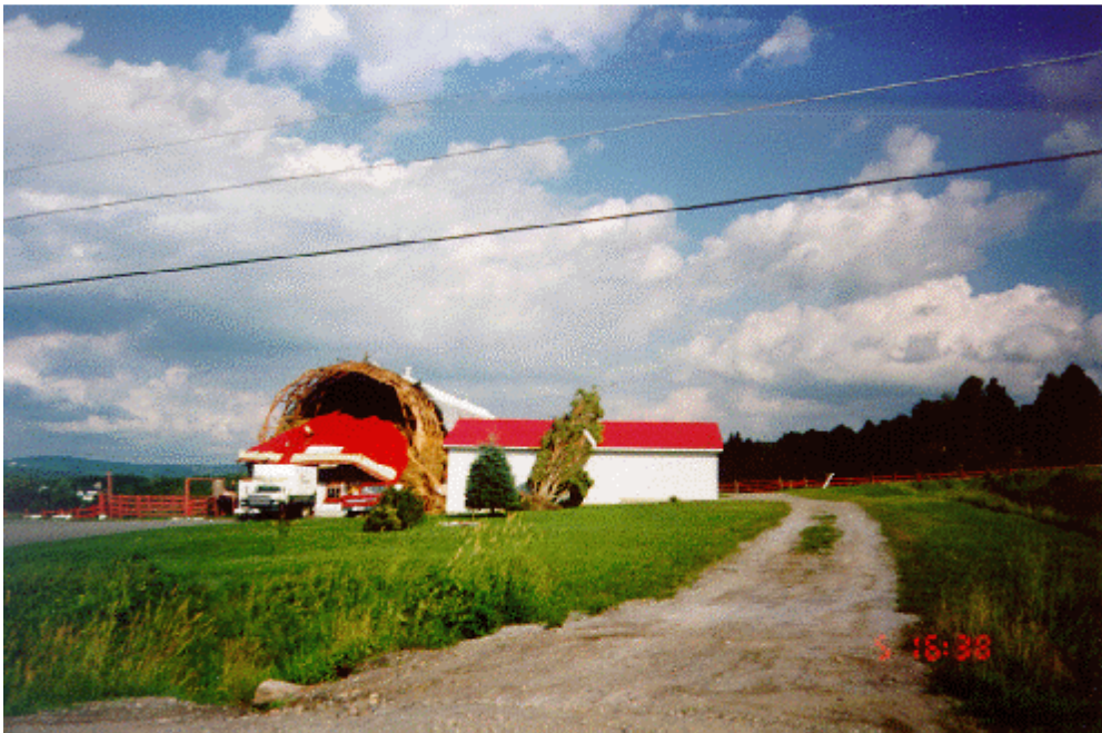
Photo 4 – West part of farm building hit by gusts near Martinville
