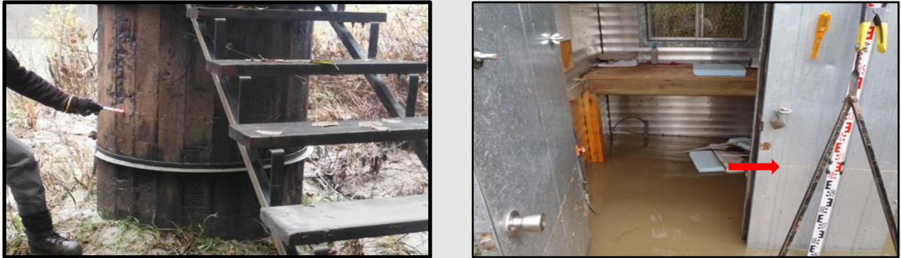
Figure 13: Examples of recording and surveying high water marks.
