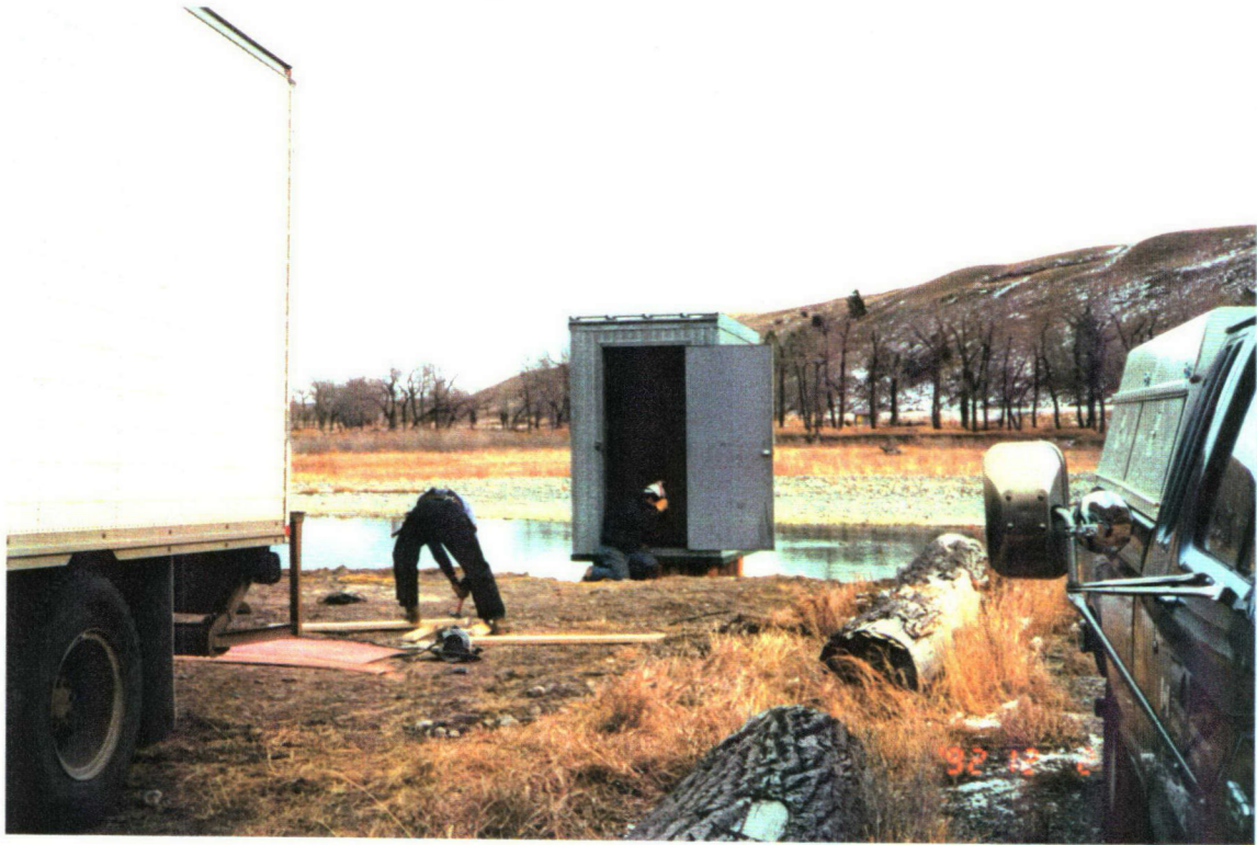
OLDMAN RIVER BELOW OLDMAN DAM COMPLETING STRUCTURE
