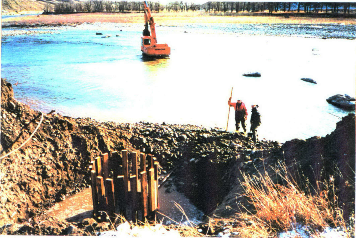
OLDMAN RIVER BELOW OLDMAN DAM EXCAVATING AND INSTALLING WELL
