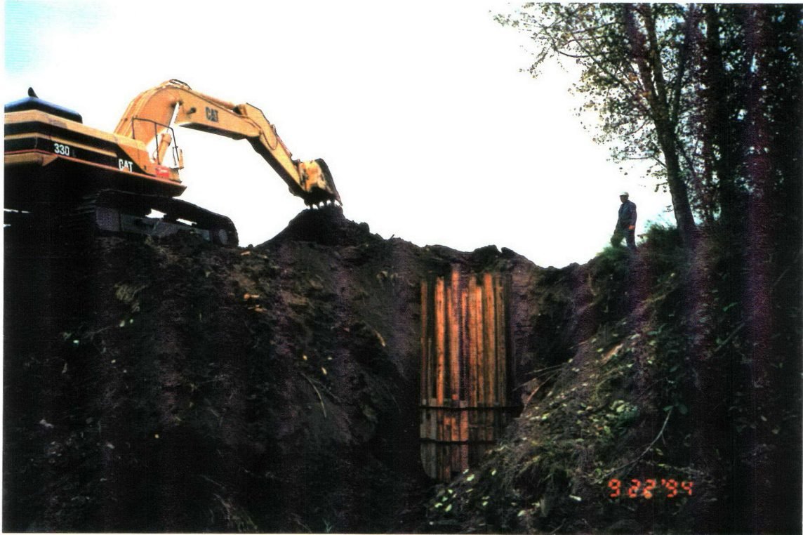
Scene's during excavating and backfilling the stilling well at the Ponton River above Boyer River 24-Sep-94
