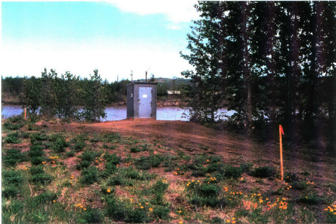
Smoky River at Watino- The Instrument shelter was dismantled and 40 yards of fill hauled in and compacted and the shelter re-installed at a higher level.
