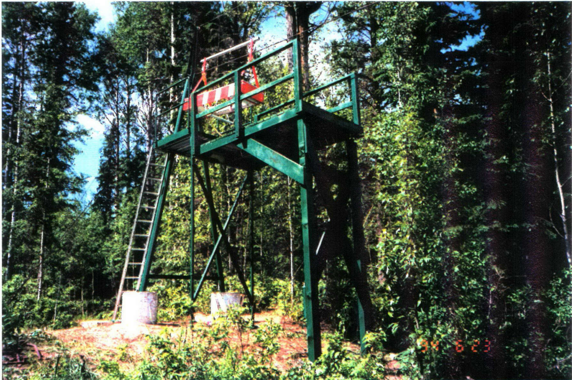
Before (Upper) and After (Lower) photo's of 18' tower replacement at the McLeod River near Whitecourt. The old wooden tower was quite rotten.
