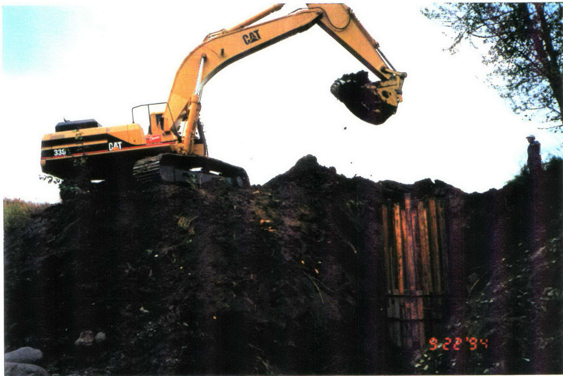
Scene's during excavating and backfilling the stilling well at the Ponton River above Boyer River 24-Sep-94
