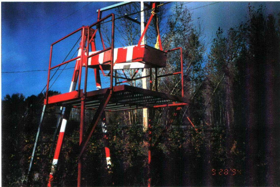
Platform extension installation at the Swan River near Kinuso.
