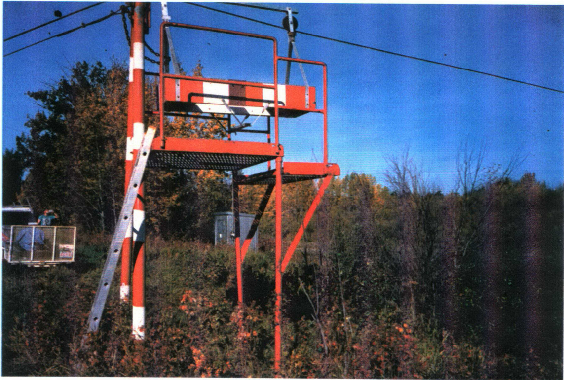
CABLEWAY PLATFORM EXTENDED AT NOTIKEWAN RIVER AT MANNING 22-SEPTEMBER-95
