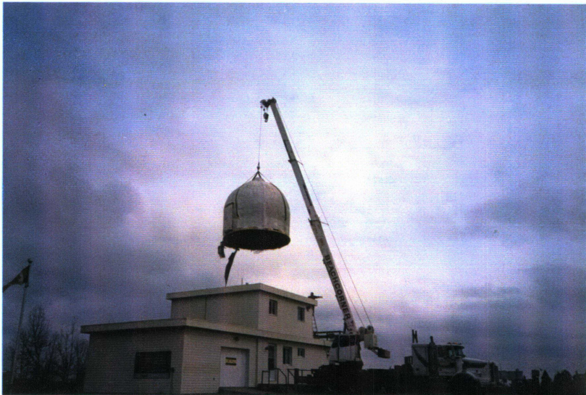
STONY PLAIN RADOME REMOVAL 17-OCTOBER-95
