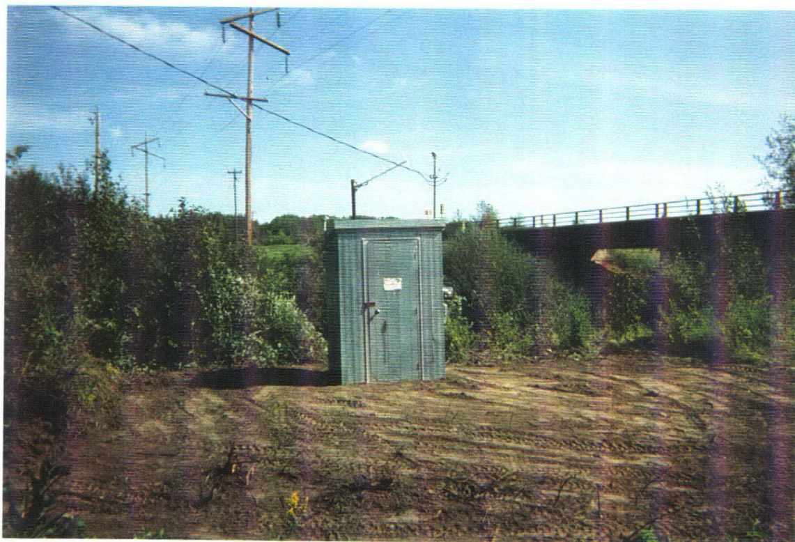
Keg River at Highway 35 (5/August/1998) Large holes had washed out around well they were backfilled and levelled.
