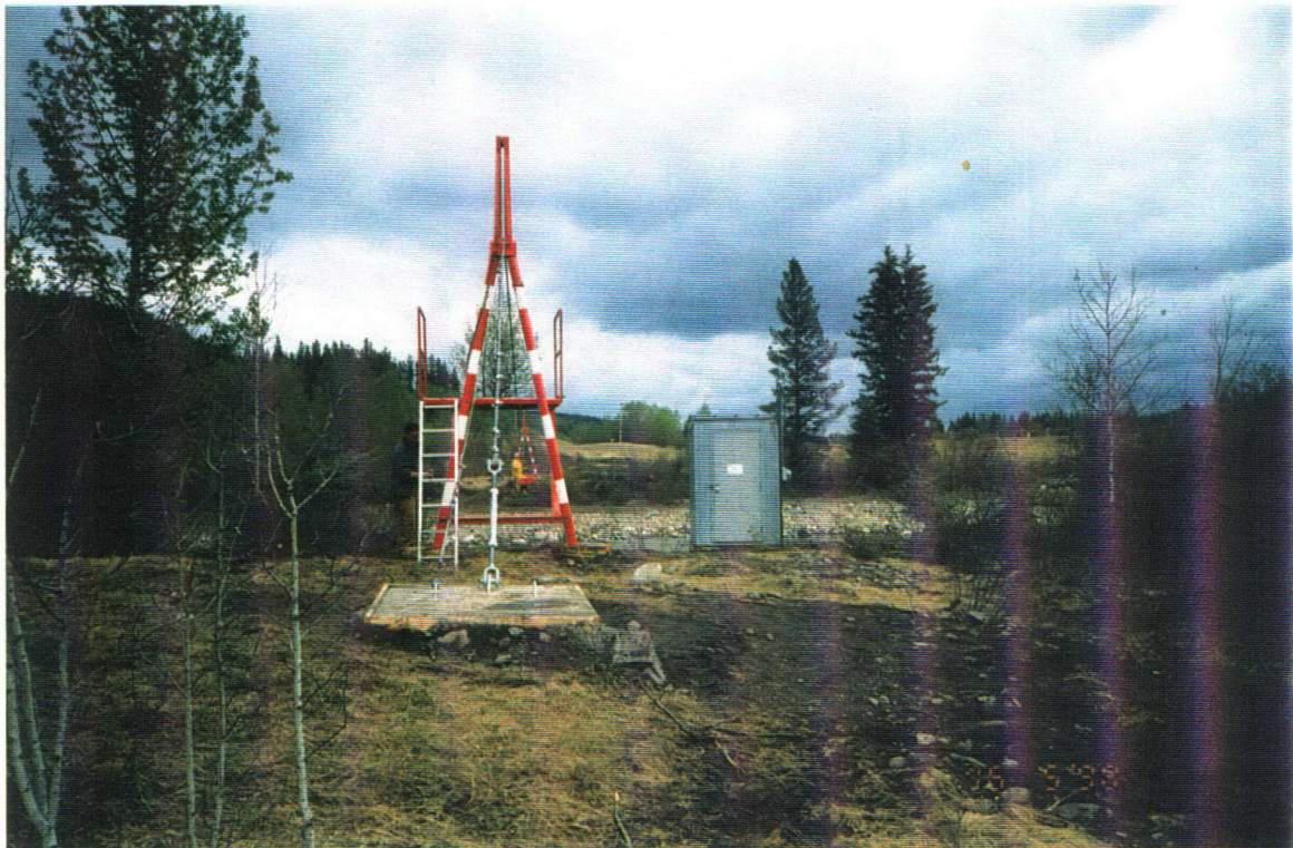
Muskeg River near Grande Cache (16/May/1998) New Cableway, Plastic well and shelter installed.
