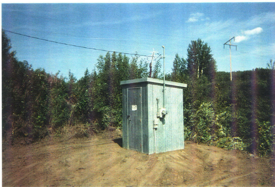
Keg River at Highway 35 (5/August/1998) Large holes had washed out around well they were backfilled and levelled.
