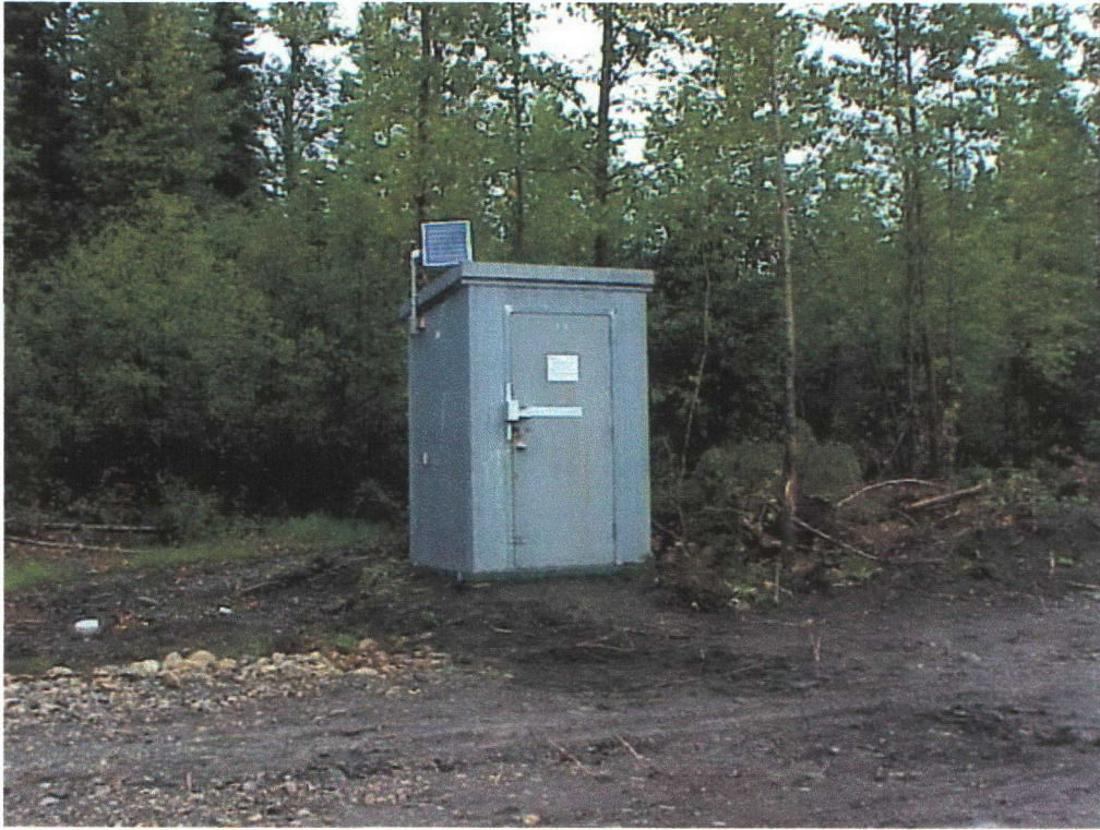
Figure 5: Ram River replacement shelter
