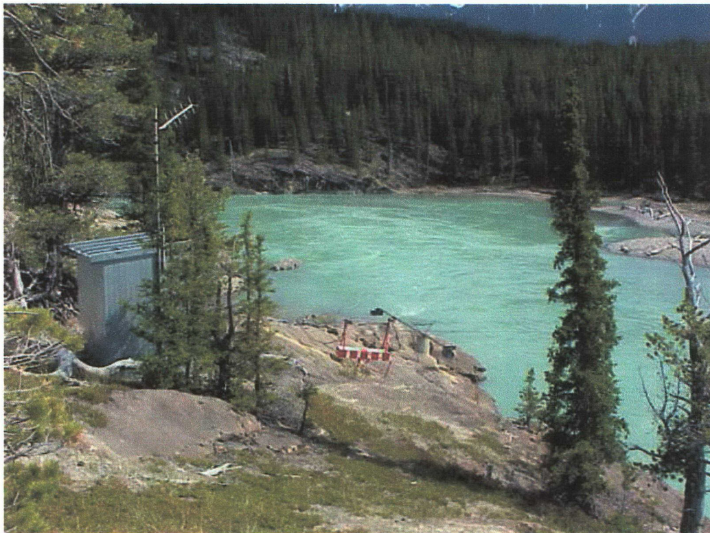
Figure 8: North Sask at Whirlpool Point Cableway project 2006/07
