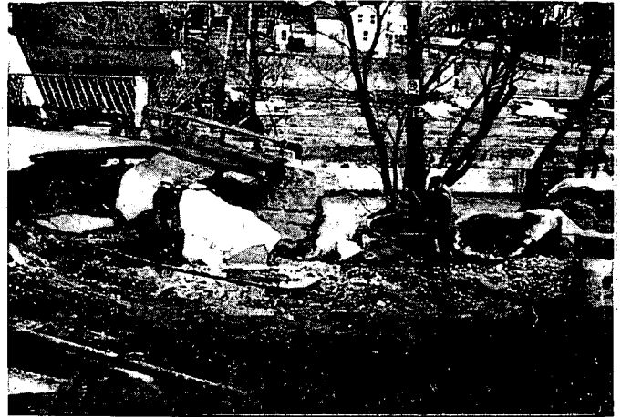
Flood damage — Ganaraska River at Port Hope
