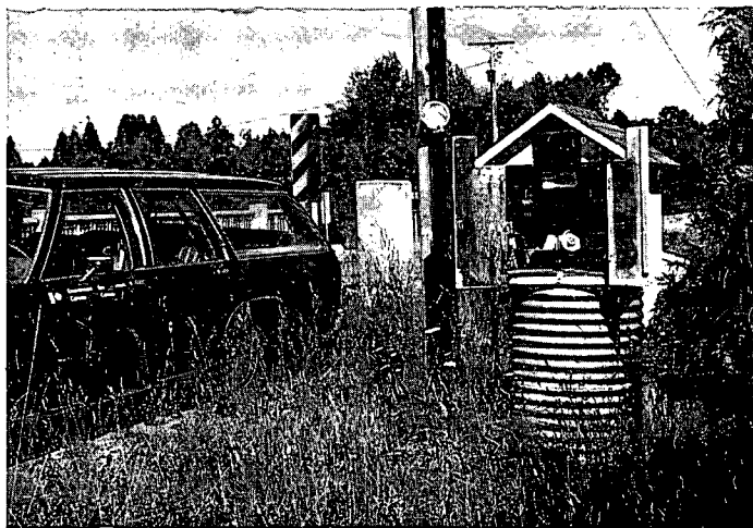
A "Guelph" Shelter housing hydrometric data measurement equipment
