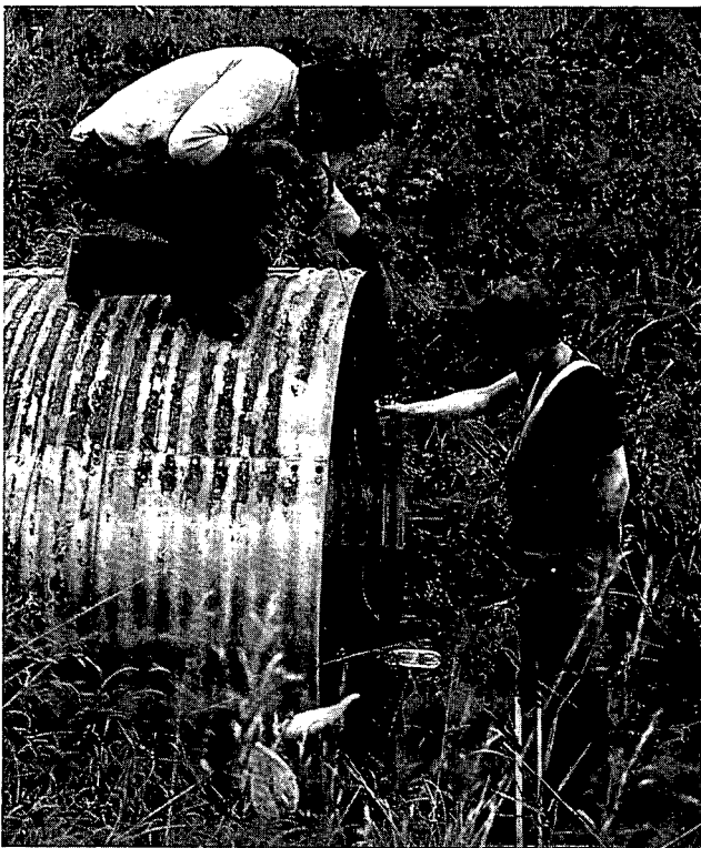
Measuring streamflow through a culvert at Oshawa Second Marsh
