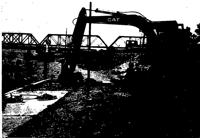
Construction at the Niagara River sampling station at Fort Erie
