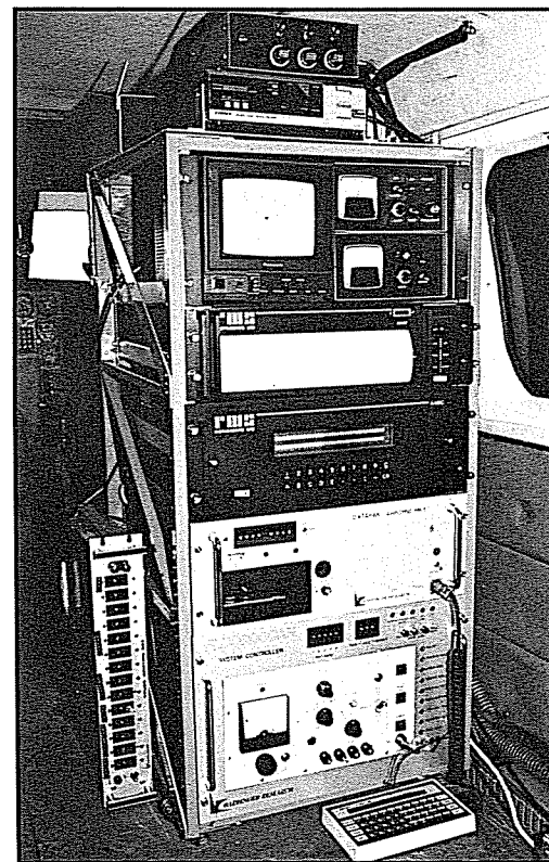
Figure 2 LEAF Operator's Console in the AeroCommander
