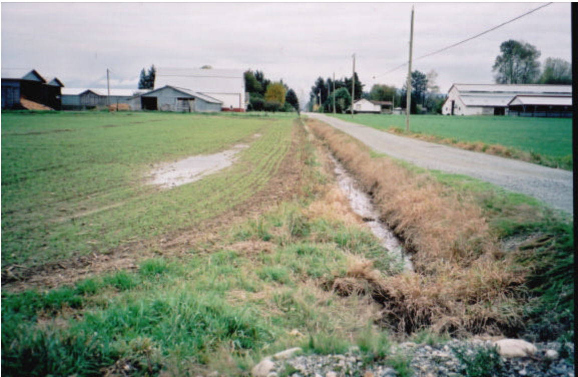
Figure 2 Sumas Road South., Chilliwack
