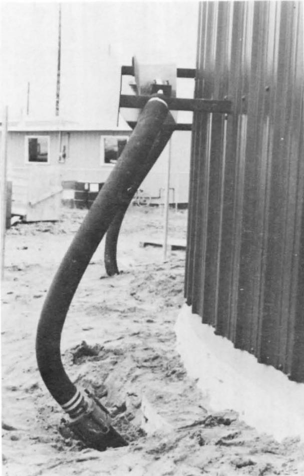
Canalisations chauffantes "Cryo-Anchors"
