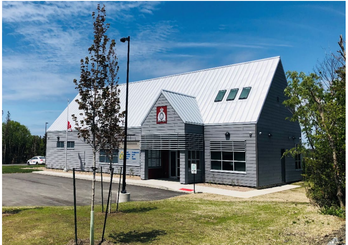
Opened in 2021, RCMP's Rocky Harbour (NL) Detachment is a Net-Zero Carbon Ready building that include state-of-the-art thermal design, automated lighting and plumbing fixtures (Photo Credit: A Simpson).
