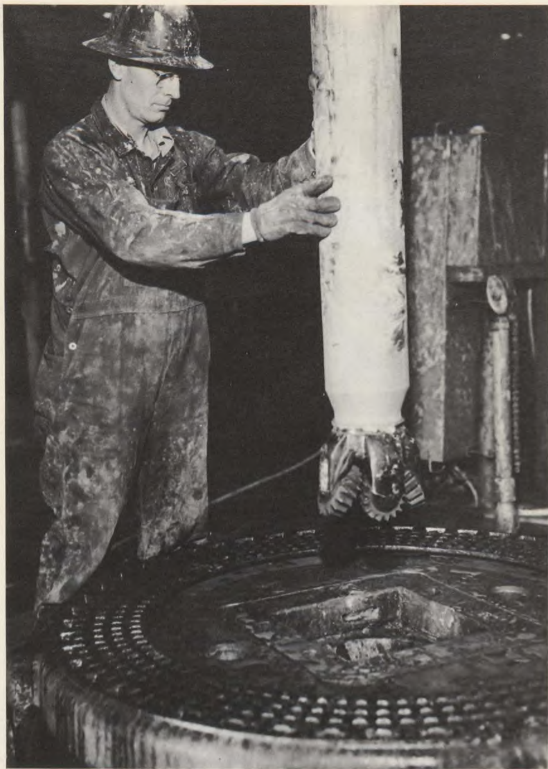
This worker is centering the drill bit before it is run down through the hole.
