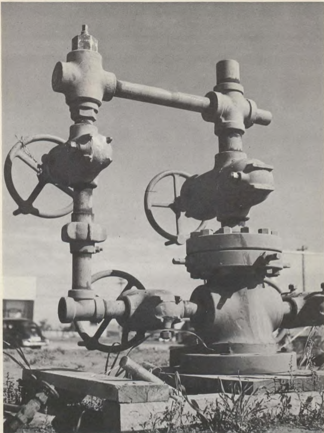
"Christmas Tree" and branching pipes are generally found on the site of capped wells once the derrick is removed.
