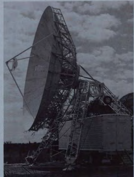
10m all-aluminum dish used for the Symphonie experiments. The 18m trailer houses the complete electronic equipment package. The antenna can be erected without mechanical aids.
