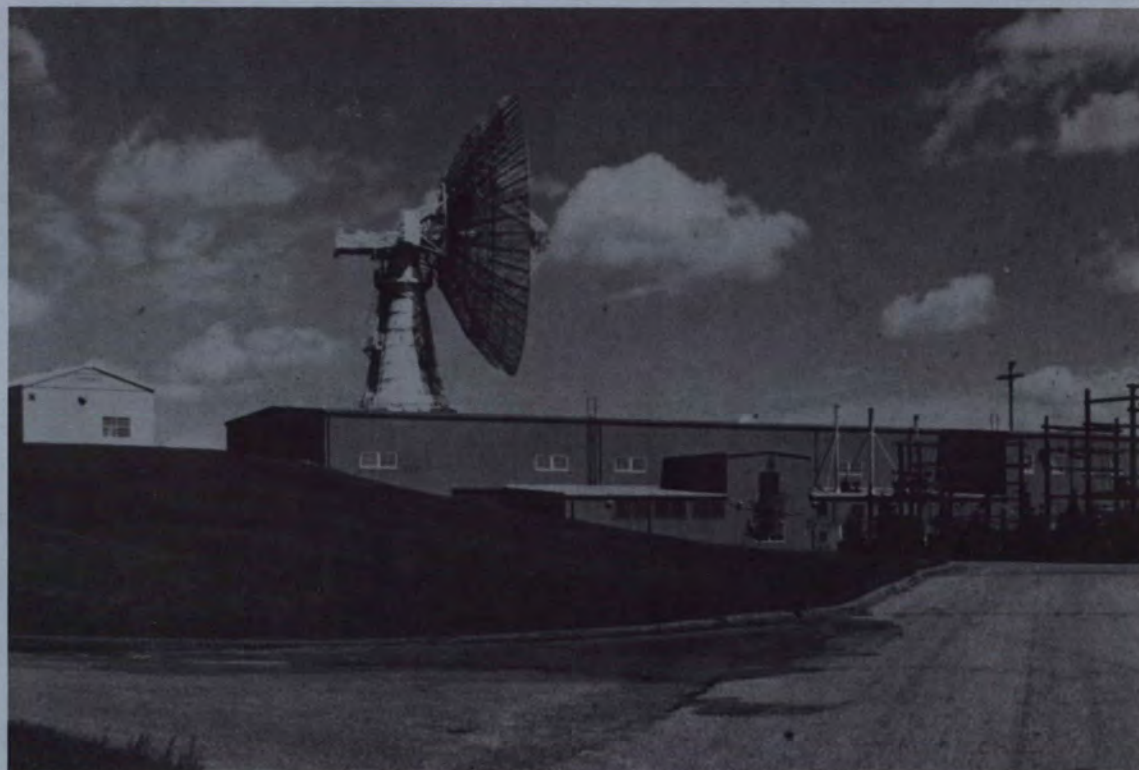
The Prince Albert satellite station records multi-spectral scanner (MSS) data from LANDSAT and very high resolution radiometer (VHRR) data from NOAA satellites. A quick look display system produces real-time images for rapid distribution to users.
