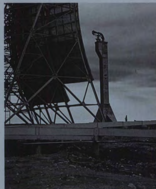
Andrew provided the 12 dual polarized one-GHz feed horns and waveguide systems for the world's first troposcatter system, reaching from Goose Bay, Labrador to Thule, Greenland.
