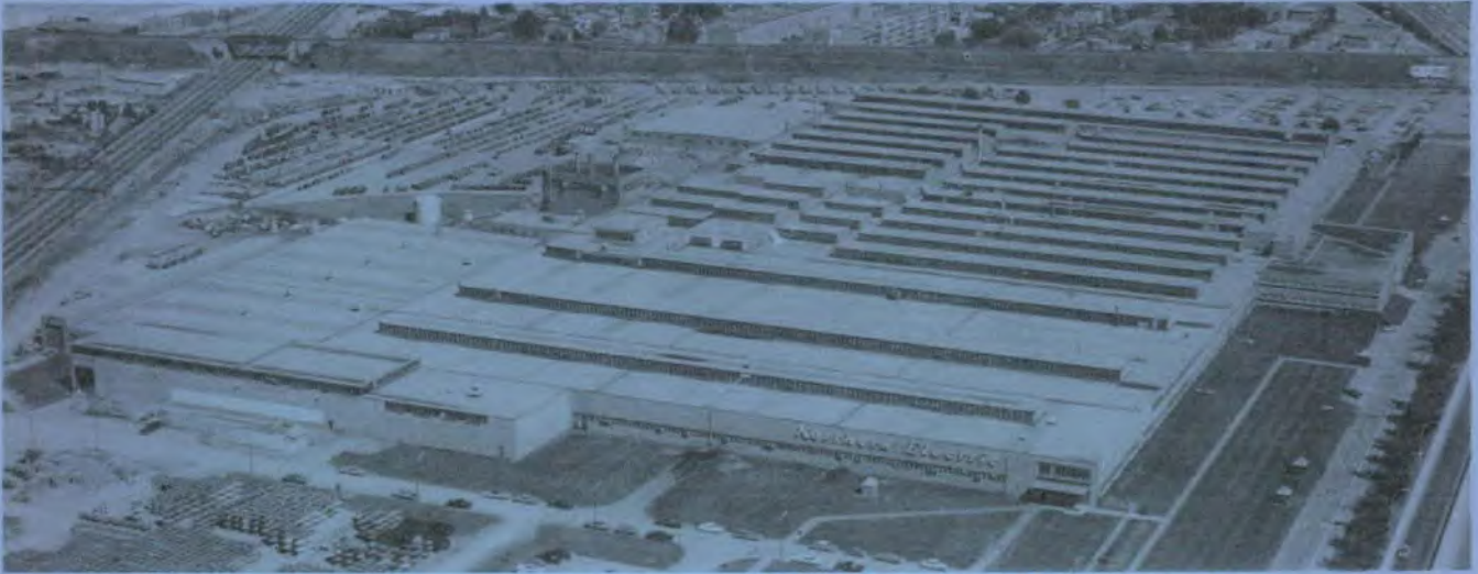
Lachine Works — Wire and Cable Lachine, Quebec
