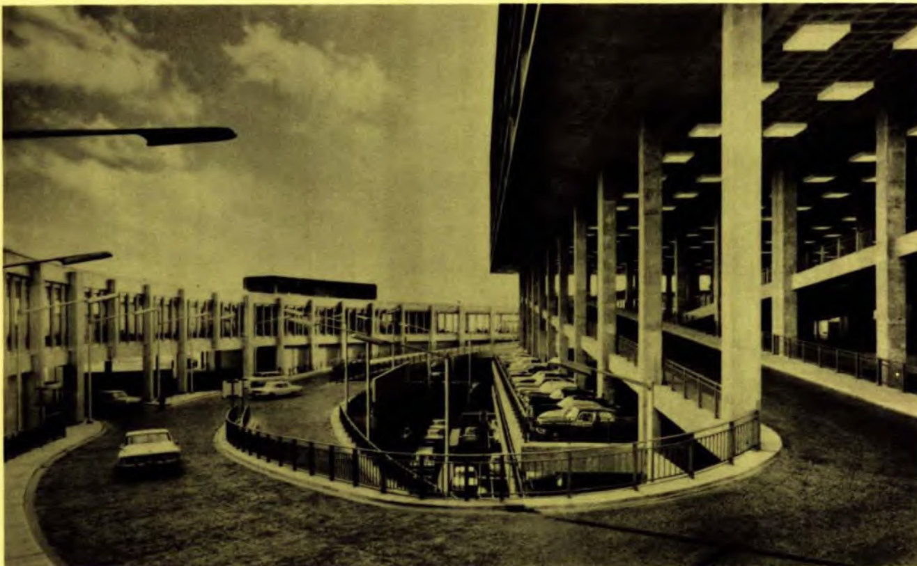
Pyrotenax MI heating cable is used to ensure snow-free roadways at all times at Toronto International Airport.
