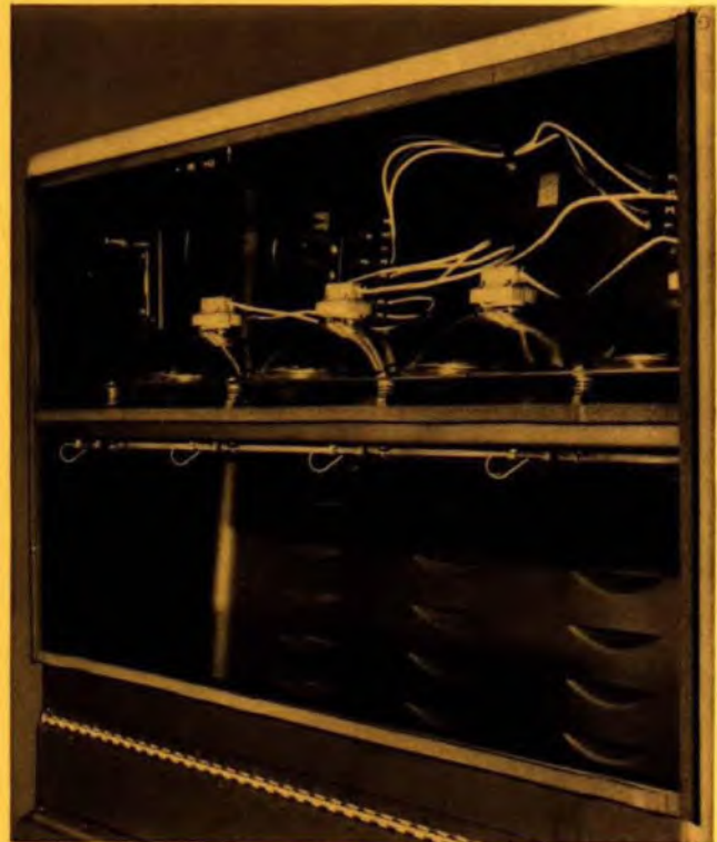
Looking down into a VASIS unit showing the four sealbeam lamp units on their adjustable spring mountings. The long vertical filters are in front of the lamp-mounting partition and held by four spring clips.
