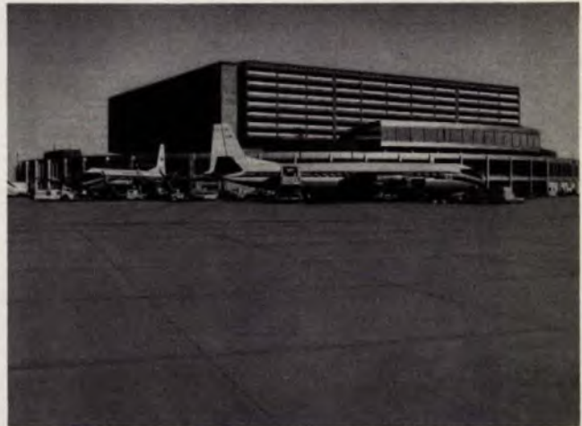
Dufferin laid sub-systems and paved the apron area of Toronto International Airport: 248,000 tons of crushed rock preceded the laying of the 83,000 cubic yards (63,457.6 M 3 ) of concrete for a 14-inch (355.6 mm) unreinforced surface with a flexural strength of 550-psi (35.15 Kg/cm 2 ) at 28 days' curing.
