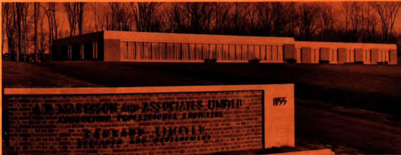
Flexibility and ease of expansion keynote the design of Margison's headquarters office building at Don Mills (Toronto).
