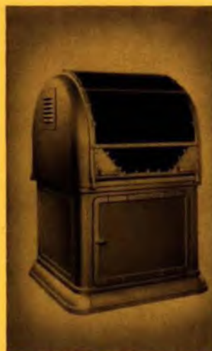
Crouse-Hinds rotating beam ceilometer projector transmits a 1,300-watt modulated light beam at the cloud base every six seconds (left).
