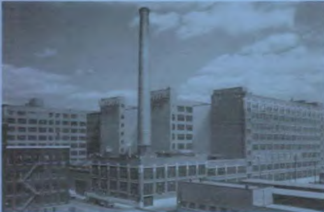
Montreal Works — Transmission Montreal, Quebec
