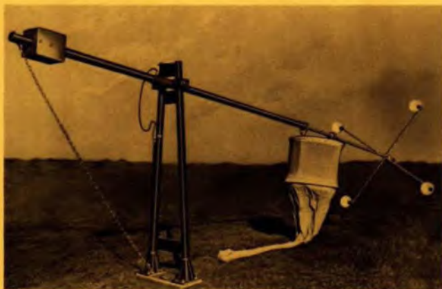
Wind cone fixture in position for servicing. Concrete balance weight is about 510 pounds (231.3 Kg) and measures 12 by 24 by 20 inches (304.8 by 609.6 by 508.0 mm)
