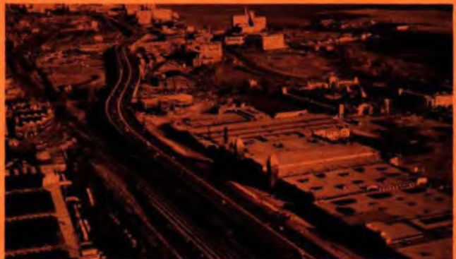
The six-lane Frederick G. Gardiner Expressway, Toronto, Ontario.
