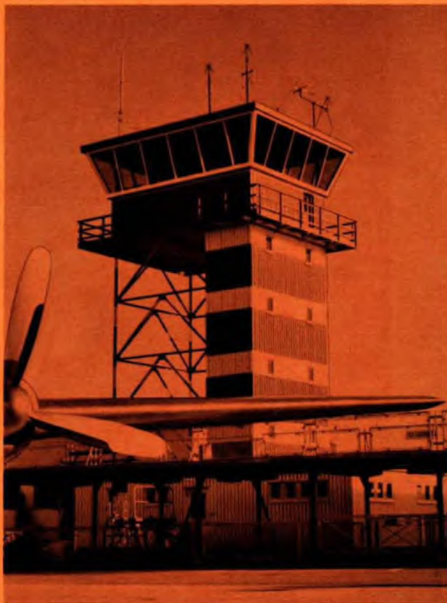
Typical airport control tower and communication antennas designed and erected in consultation with Hoyles, Niblock and Associates.
