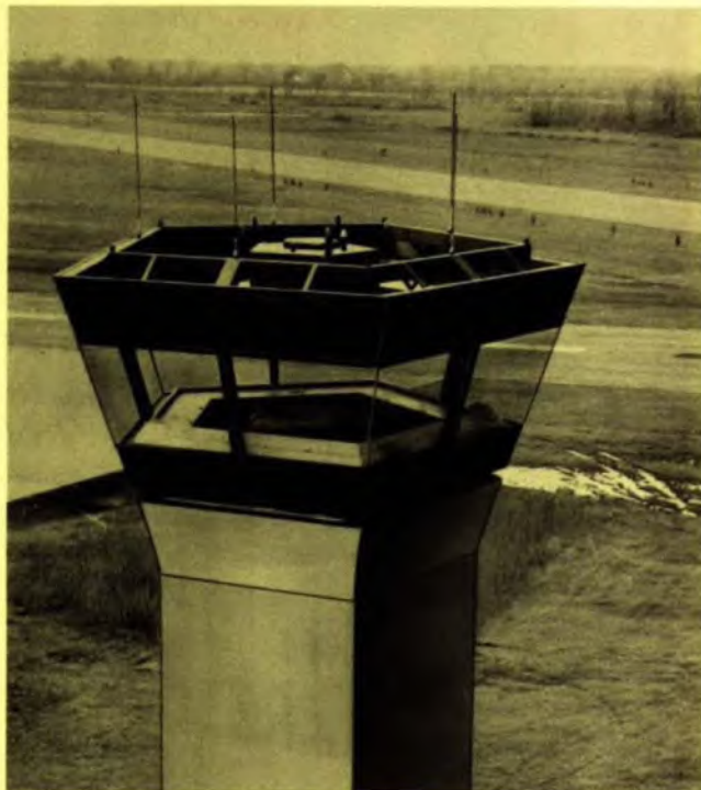
Canadair Limited's air traffic control tower cab is an ultra-modern unit which will accommodate every facility for air traffic control. It is prefabricated and finished for on-site assembly and includes a full range of modular modules. The 275 square feet (25.5 square metres) of floor area provides adequate space for four men.
