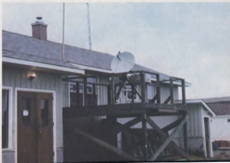
(d) Telephony terminal with 1 m diameter antenna at Kashechewan, Ontario.
