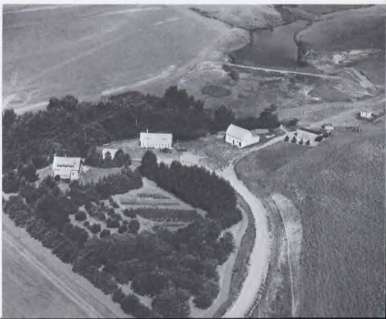
This small dam impounds a dependable water supply for stock-watering, farmstead irrigation and domestic use.
