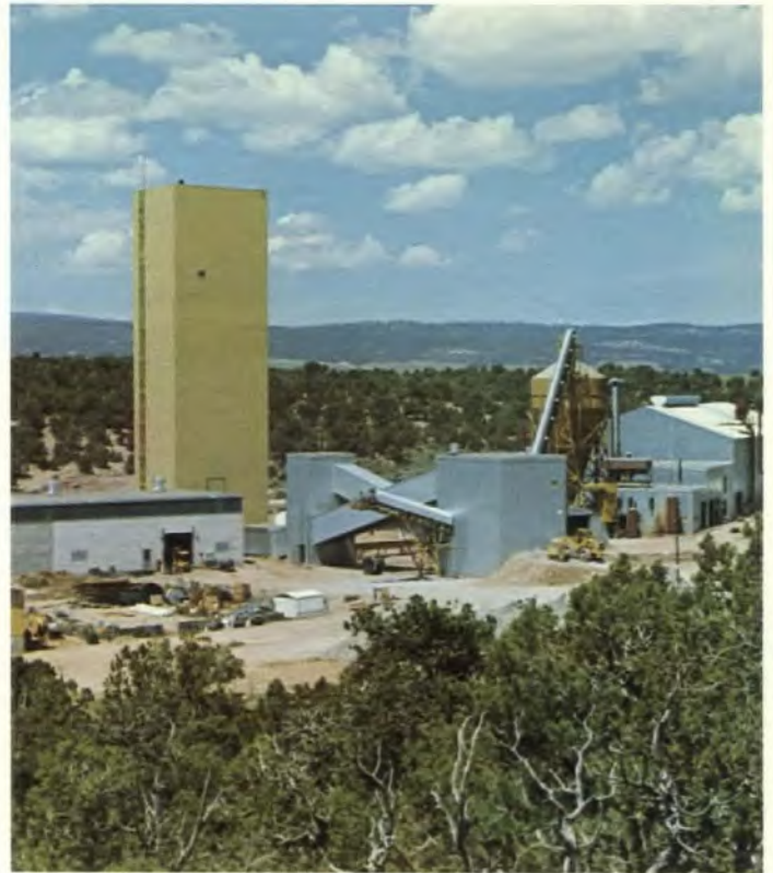
500 ton per day uranium concentrator engineered for Rio Algom Limited at Moab, Utah.
