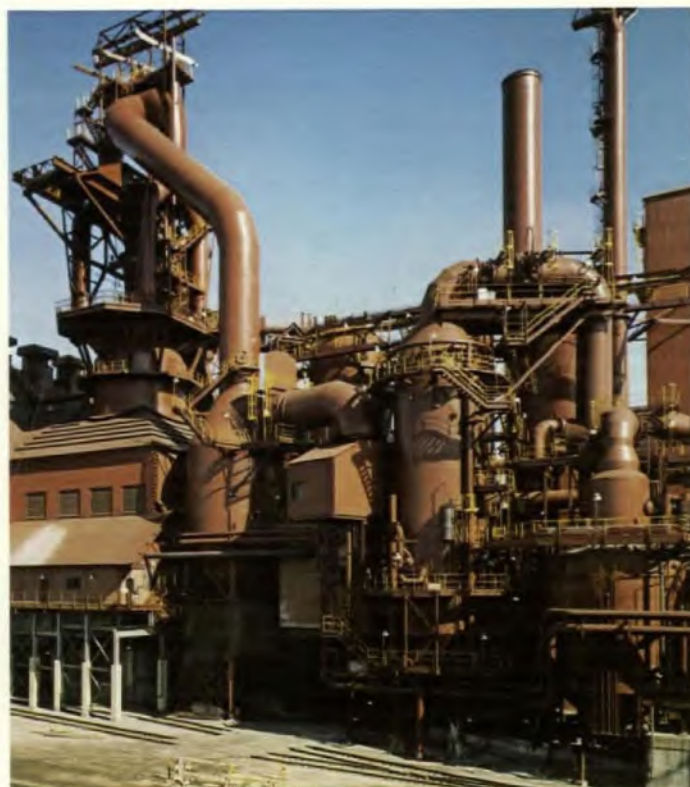
#4 blast furnace and ancillaries, computer controlled operation and modern environmental controls provide efficient operation of this 4000 tons per day blast furnace engineered and constructed for Dominion Foundries and Steel Limited at Hamilton, Ontario.
