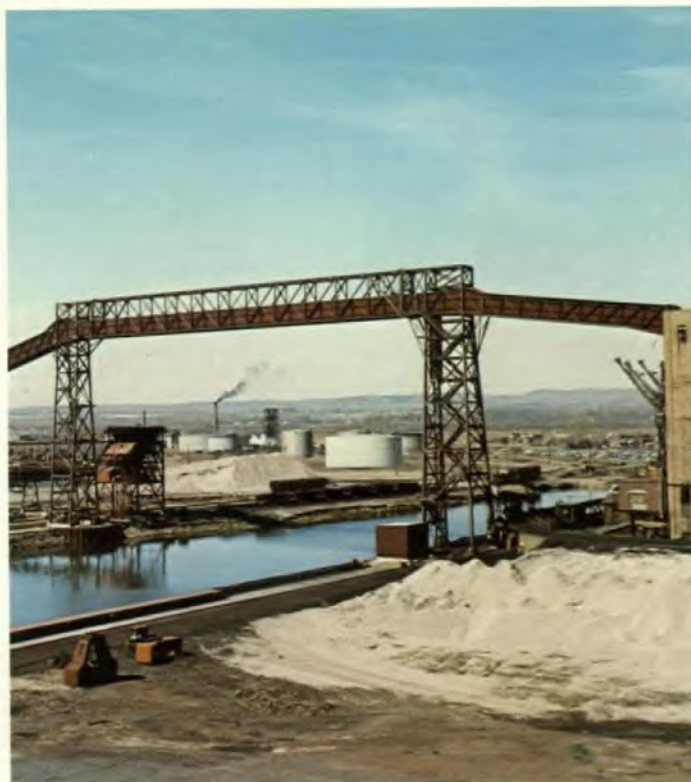
Conveyor bridge over the docking slip forms part of a coal stocking out and reclaim facility, designed and constructed for The Algoma Steel Corporation at Sault Ste. Marie, Ontario.
