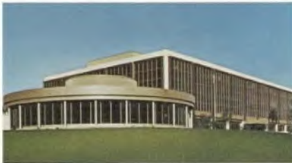
B. Extension of Otto Main Offices, Bochum, West Germany
