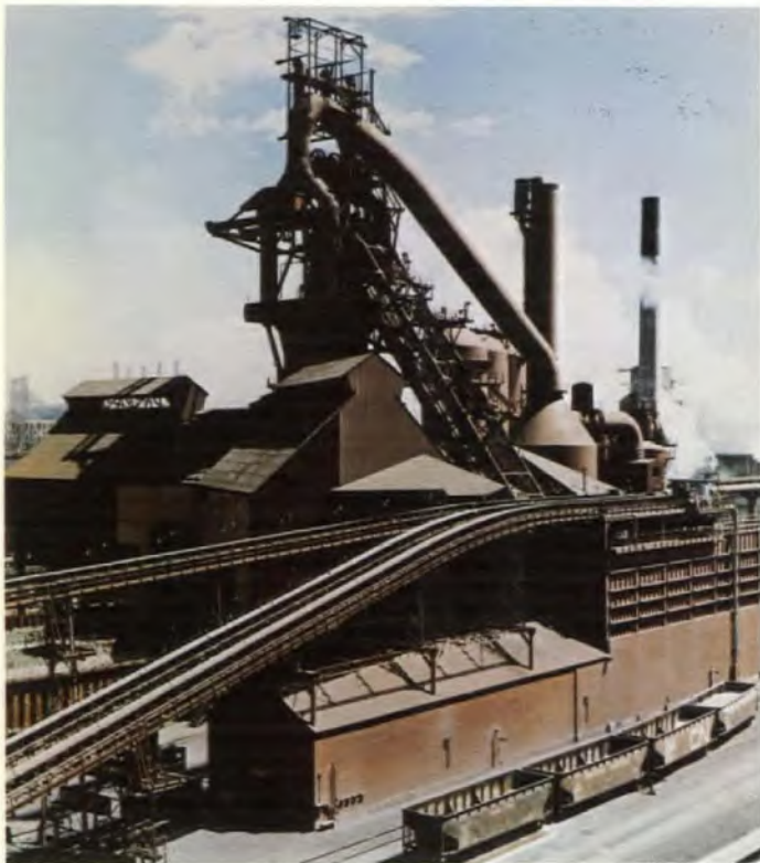
"E" blast furnace — largest blast furnace in Canada at the time having a capacity of 3500 tons of iron per day with provision for expansion to 5000 tons per day. One of 3 blast furnaces designed and built for The Steel Company of Canada Limited at Hamilton, Ontario.
