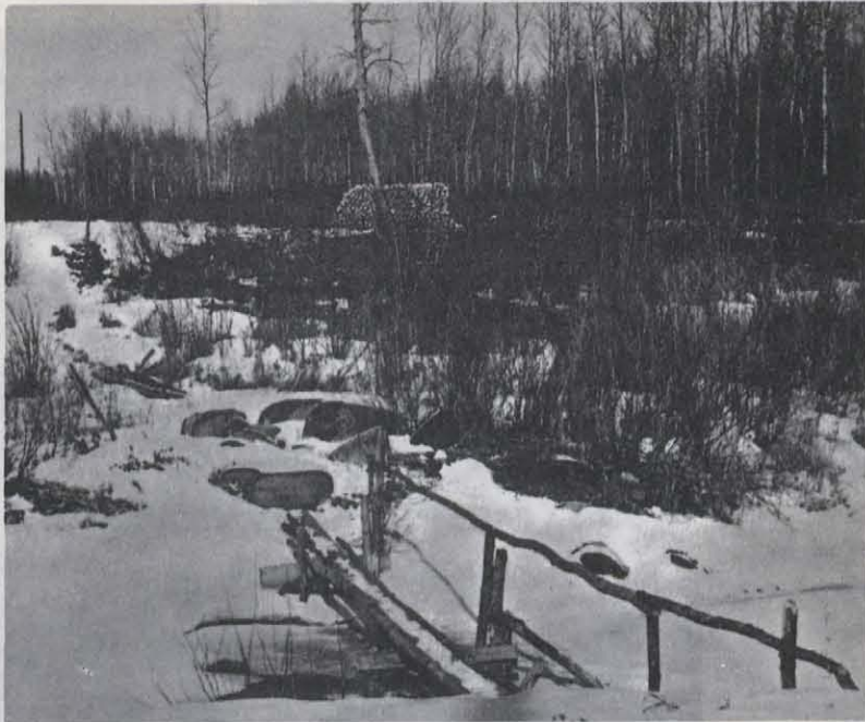
A footbridge over Fisher River
