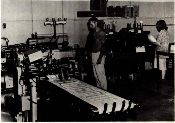
This automatic bindery equipment, installed by Kentville Publishing Co. Ltd. with the assistance of Area Development grants, accepts signatures printed and folded on a web offset press, assembles, stitches and trims them with a maximum capacity of 10,000 booklets per hour.
