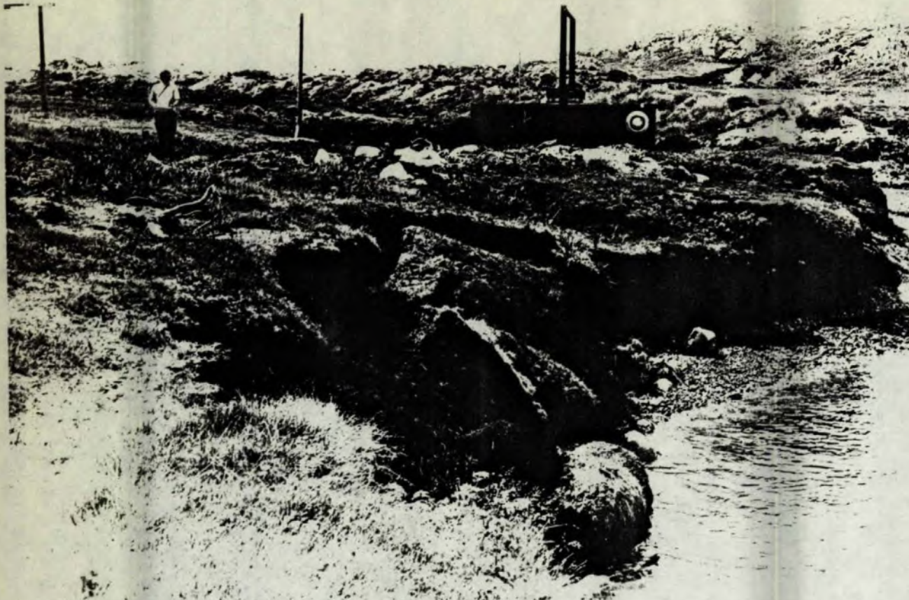
PHOTO NO. 4 Close-up of bog erosion at Island Cove. The edge of bog is only 15 feet from the pipeline at this point.
