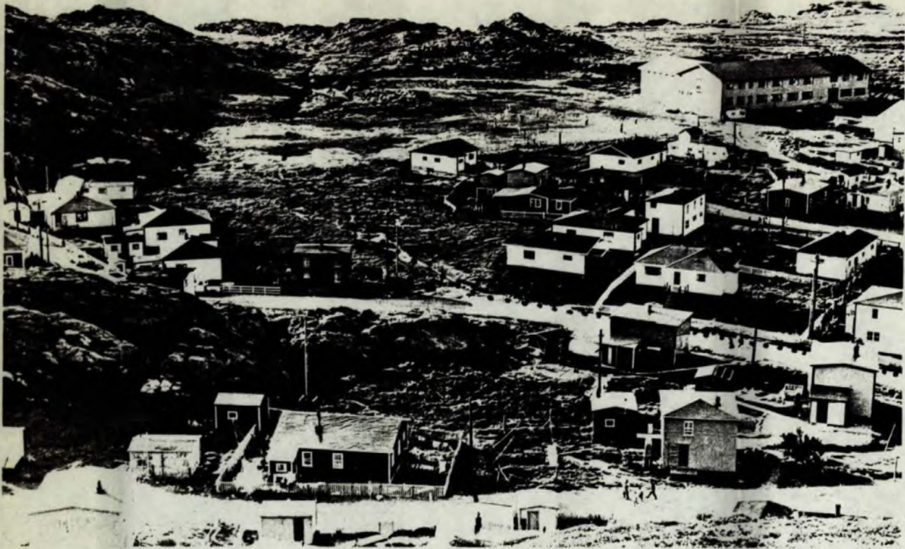
PHOTO NO. 1 General view of pipeline route through bog area and school yard.
