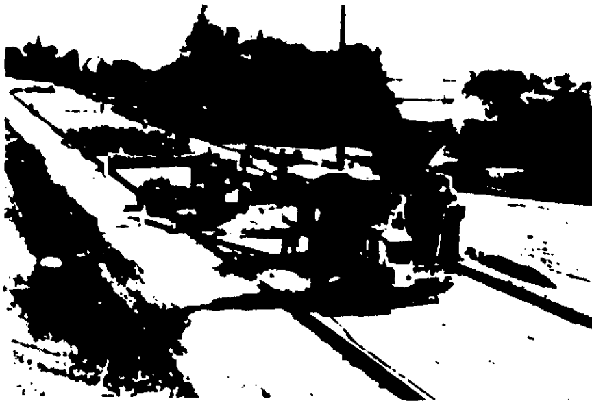
Fig. 19. Paving mixer in operation.
