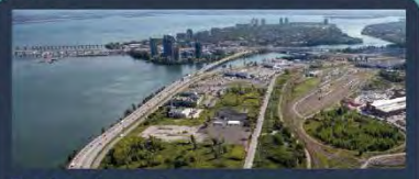
Federal section of Bonaventure Expressway
