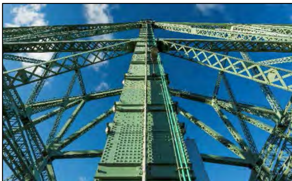
Superstructure of the Jacques Cartier Bridge
