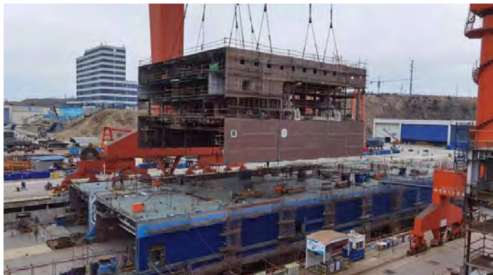
Accommodation blocks lifted onto the new vessel.
