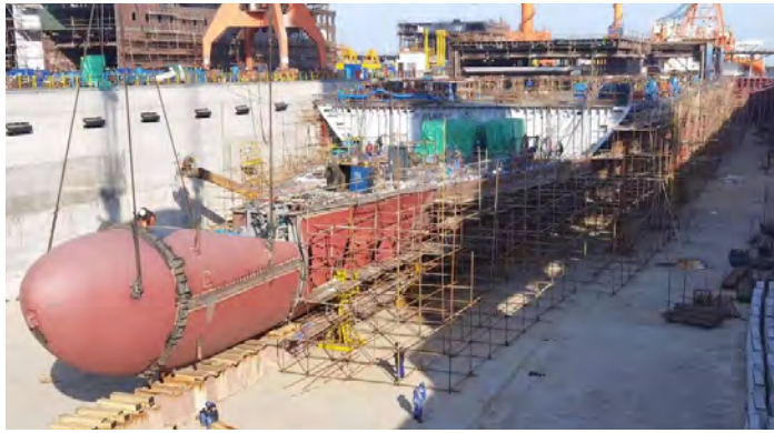
Accommodation blocks lifted onto the new vessel.
