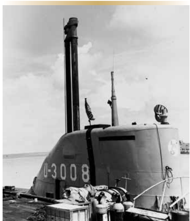
The surrendered Type-XXI U-3008 at Key West, Florida. The USN studied U-boat snorkel designs after the war for their own submarine programs.
