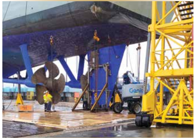
Figure 11. Charlottetown rudder installation.
