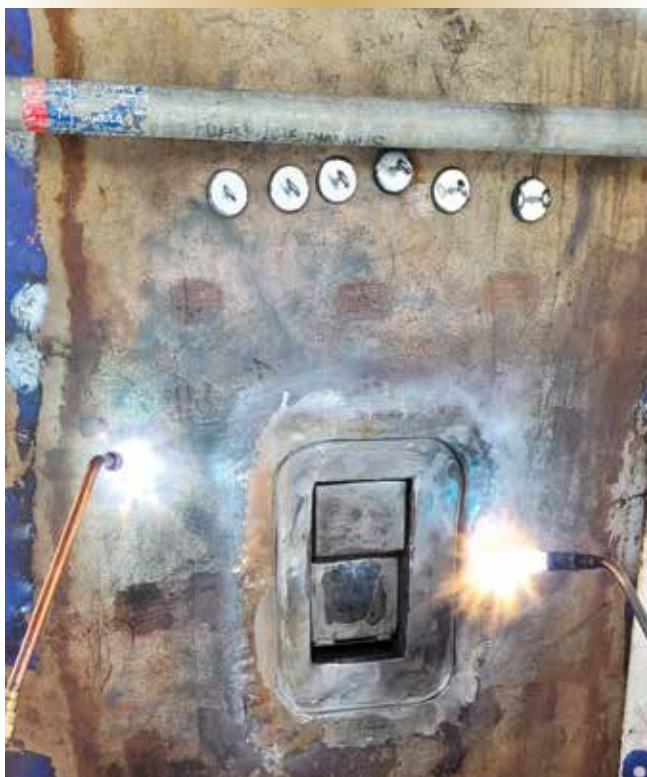
Figure 10. Pre-heating Charlottetown's rudder hub casting prior to welding the securing wedges in place.
