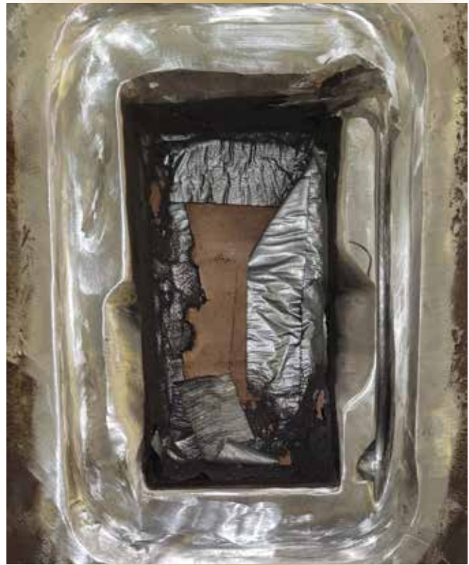
Figure 8. Charlottetown's temporary keyway window repair with defects removed.
