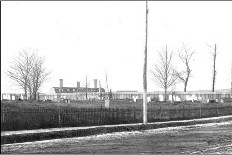
FIGURE 4. A BOARD FENCE SEPARATES THE GRAVEYARD FROM THE FORT GROUNDS, LATE 1800s
