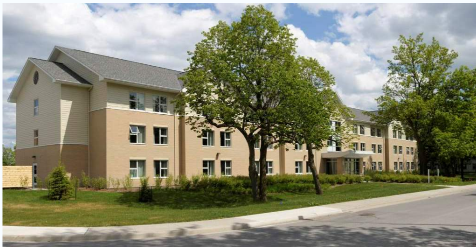
The new $12 Million Vimy Training Quarters at CFB Kingston, is a three-storey, 5,160 square metre military residence, and a model of energy efficiency and sustainable design. Built to be green, the new building includes a number of features to reduce energy consumption.
