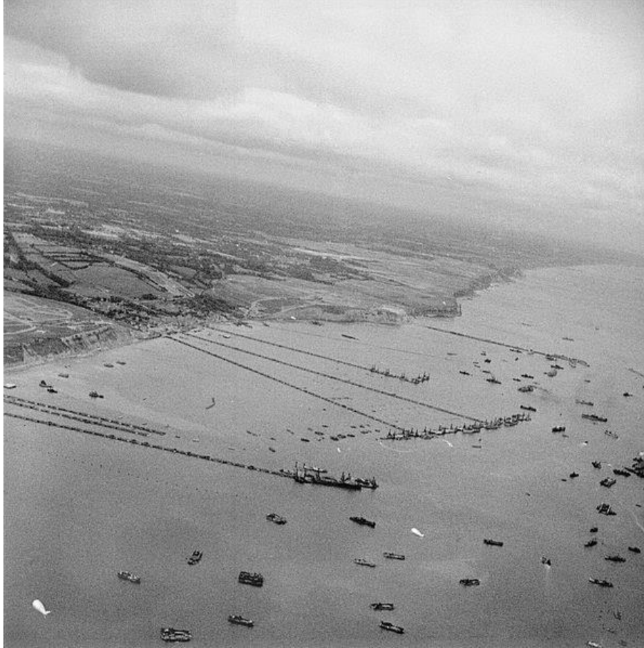
21 - An aerial oblique photograph of the Mulberry Harbour off Arromanches-les-Bains. Artificial harbours were constructed along the beach shortly after D-Day so that armoured vehicles and heavy guns could be landed. Source: http://media.iwm.org.uk/iwm/mediaLib/8/media-8246/large.jpg 1
