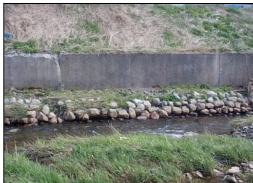
Figure 39. Rip rap lined along a section of walled stream bank
