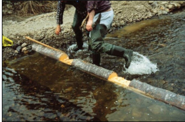
Figure 31. Installing the transversal beam across the stream bed
