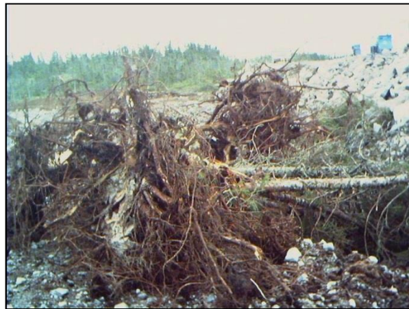
Figure 34. Typical rootwad bundles prior to placement
