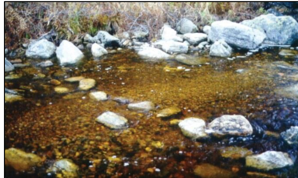
Figure 51. Gravels placed upstream of a loose boulder cluster
