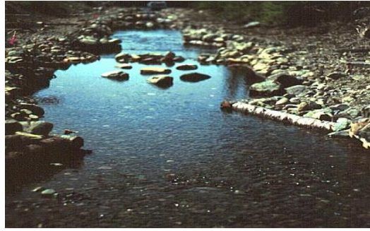
Figure 43. Example of single wing deflector
