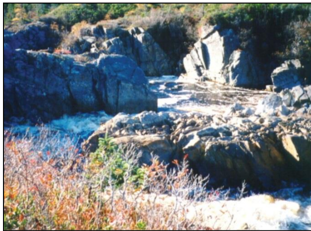
Figure 56. Blasted side channel around existing barrier to migration
