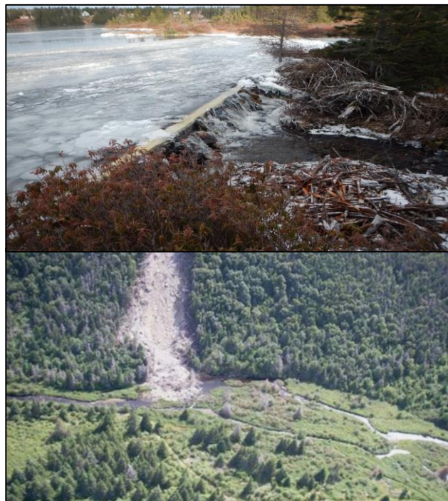
Figure 13. Top photo: a man-made dam causing obstruction at pond outflow. Bottom: Landslide causing obstruction of stream
