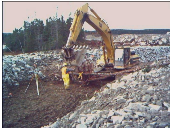
Figure 54. Construction of man-made riffle pool sequences
