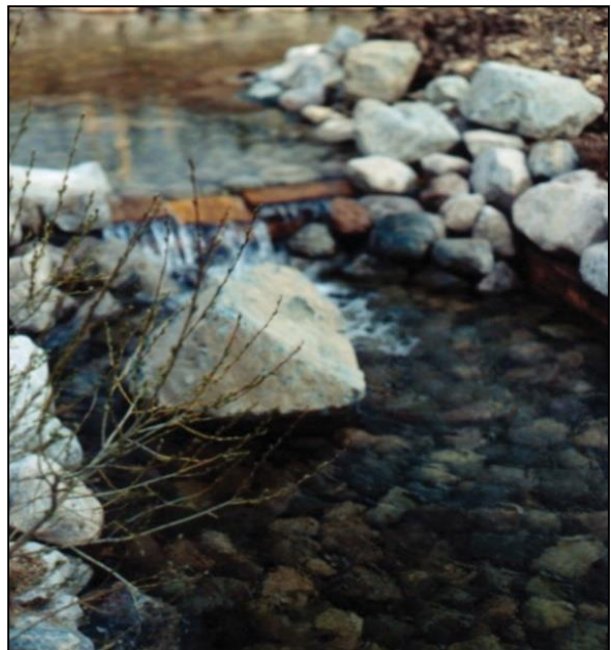
Figure 30. Properly installed wooden low head barrier
