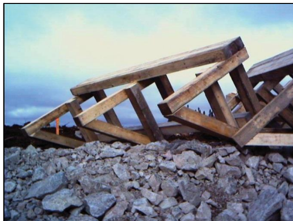
Figure 35. Prefabricated frame made of wood for undercut bank treatment
