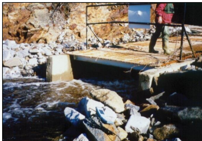
Figure 55. Outflow of typical vertical slot fishway
