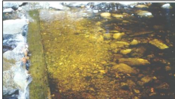
Figure 50. Gravels accumulating at the upstream end of a low head barrier
