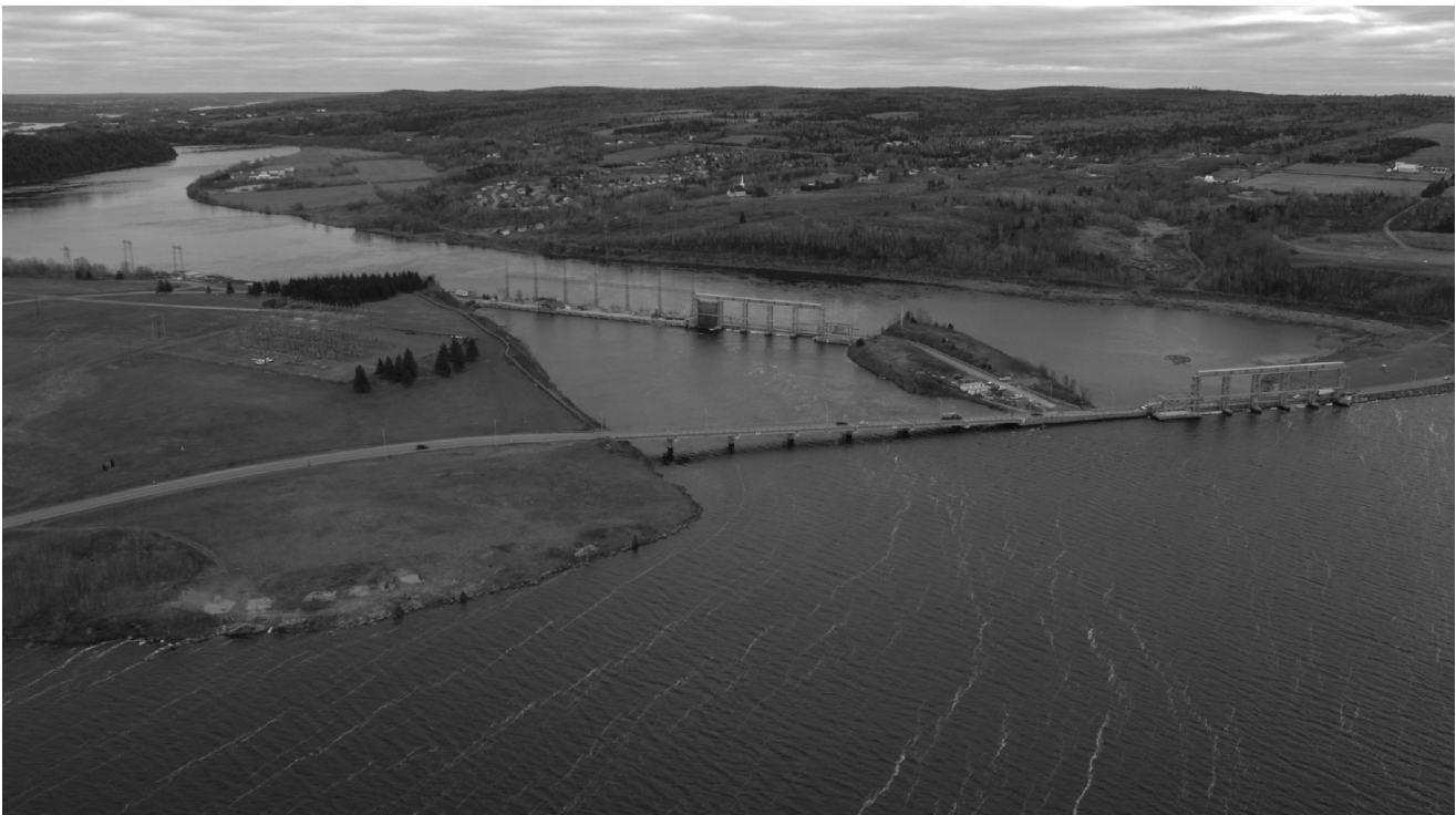
MACTAQUAC DAM — FROM THE WEST (2006)
