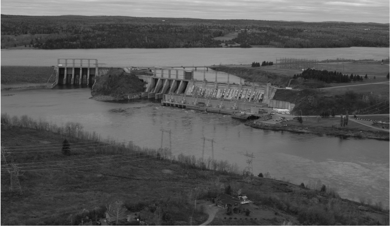
MACTAQUAC DAM — FROM THE EAST (2006)
