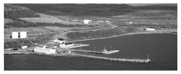
a small breakwater constructed of boulders creating a basin for small boats with an entrance width of 23 feet (7 m) and a least depth of 4 feet (1.1 m) in the entrance. Floating docks are moored in the basin. A slipway is located alongside the basin.
