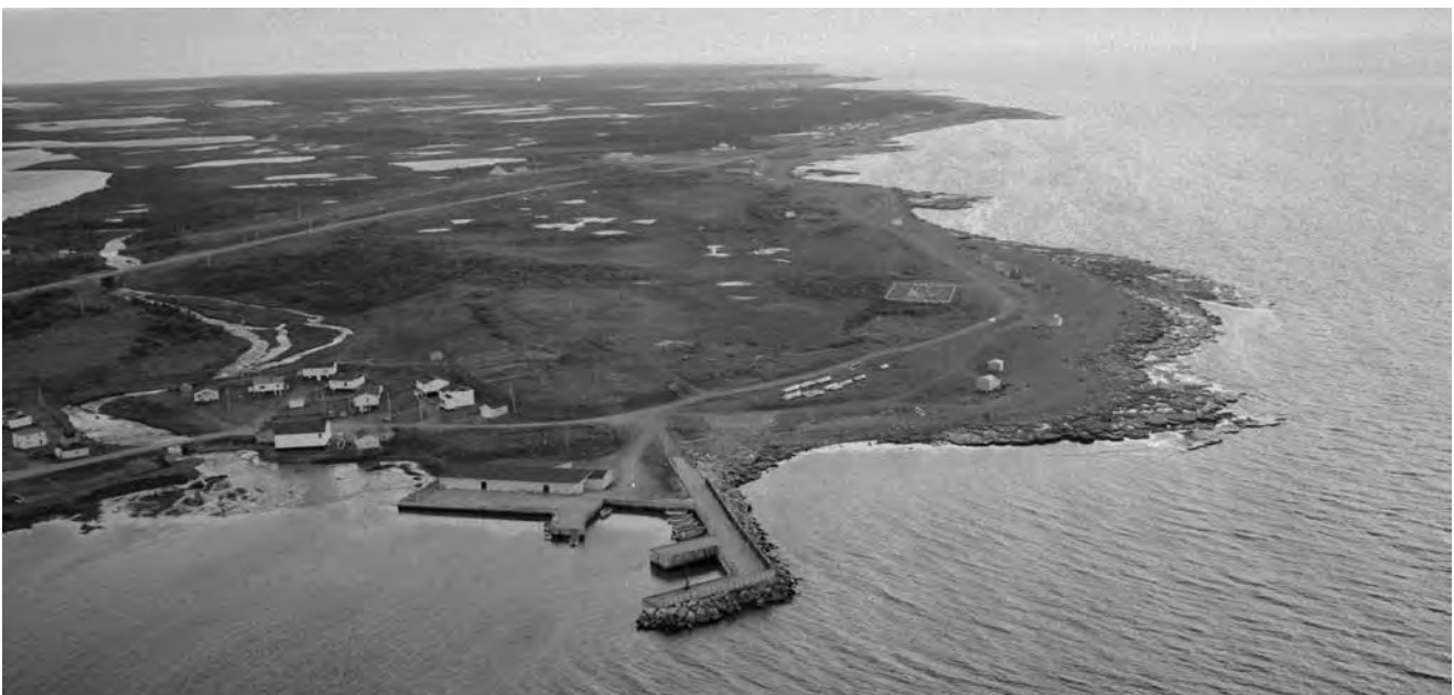
GREEN ISLAND BROOK PUBLIC WHARF (2001)
