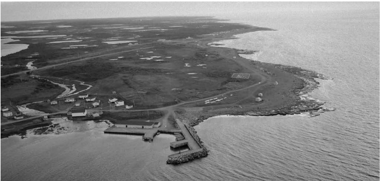
GREEN ISLAND BROOK PUBLIC WHARF (2001)
