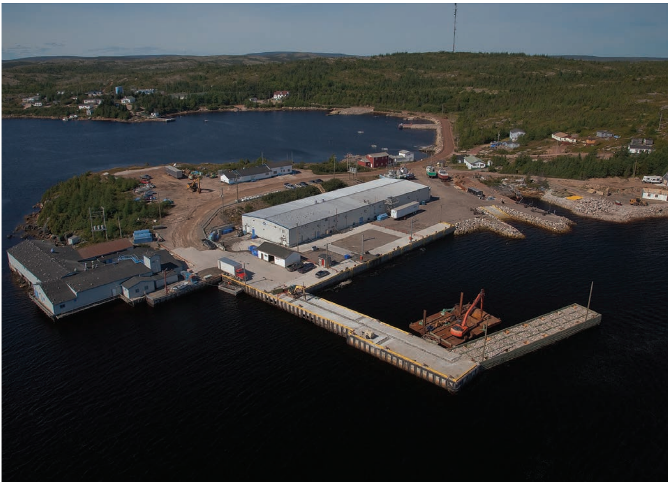
MARY'S HARBOUR PUBLIC WHARF (2015)
