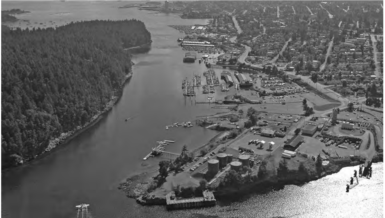
NEWCASTLE ISLAND PASSAGE LOOKING SE (2005)
