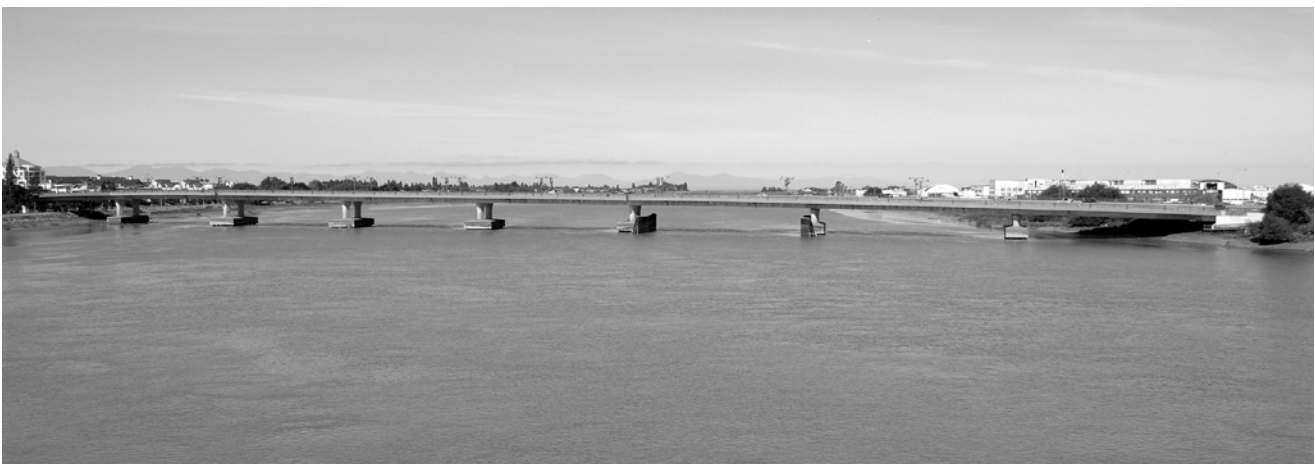
NO. 2 ROAD BRIDGE (2007)
