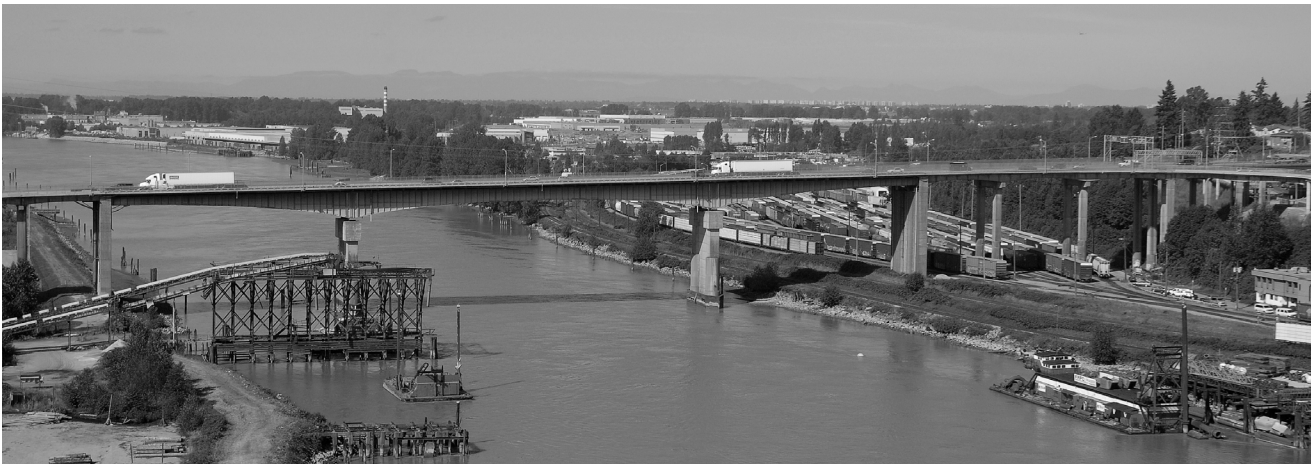
QUEENSBOROUGH HIGHWAY BRIDGE (2007)
