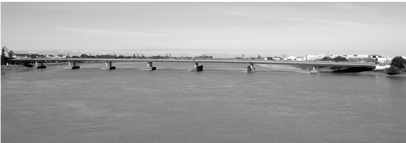
NO. 2 ROAD BRIDGE (2007)
