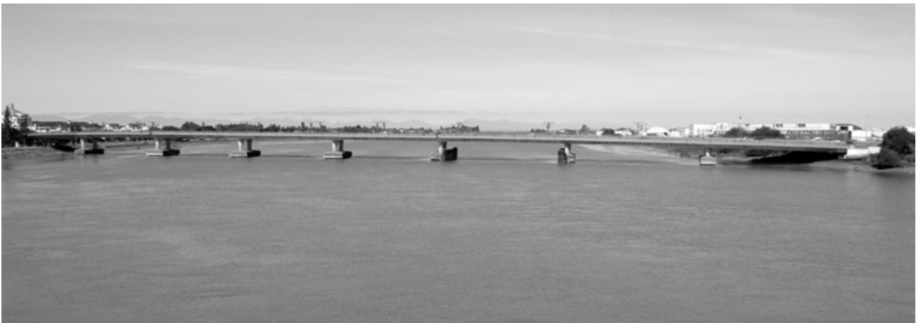
NO. 2 ROAD BRIDGE (2007)
