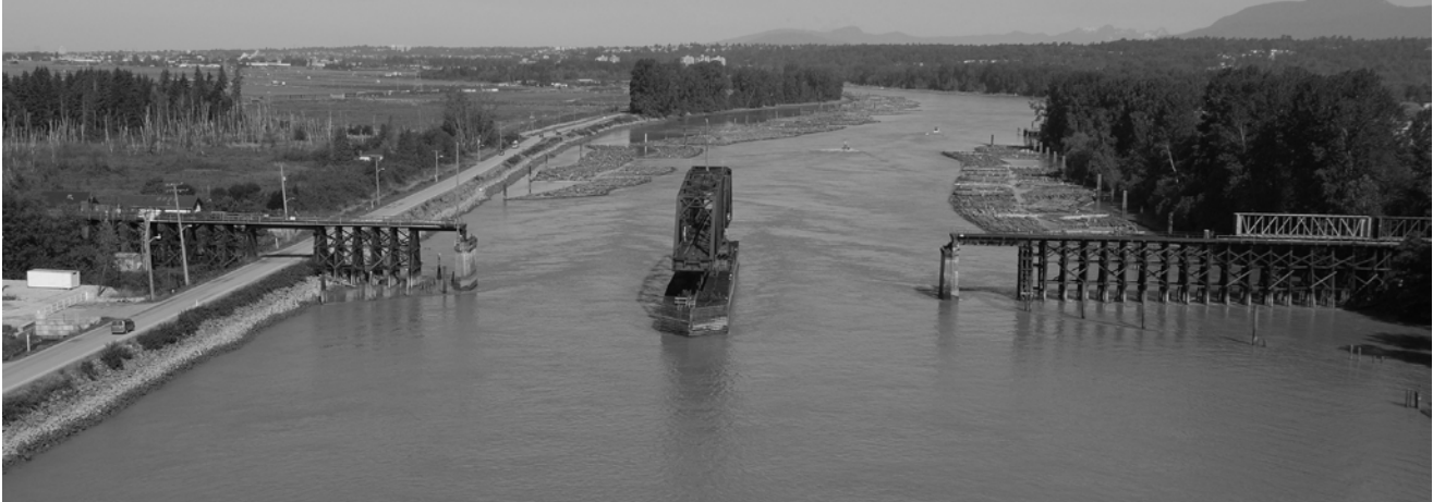
CANADIAN NATIONAL RAILWAY BRIDGE (2007)
