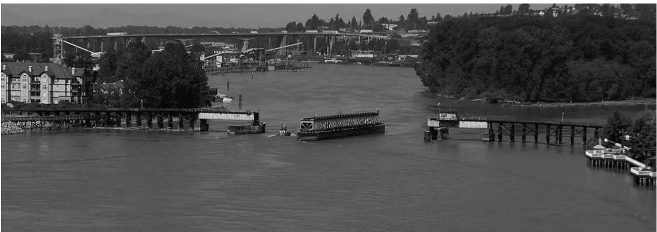
QUEENSBOROUGH RAILWAY BRIDGE (2007)
