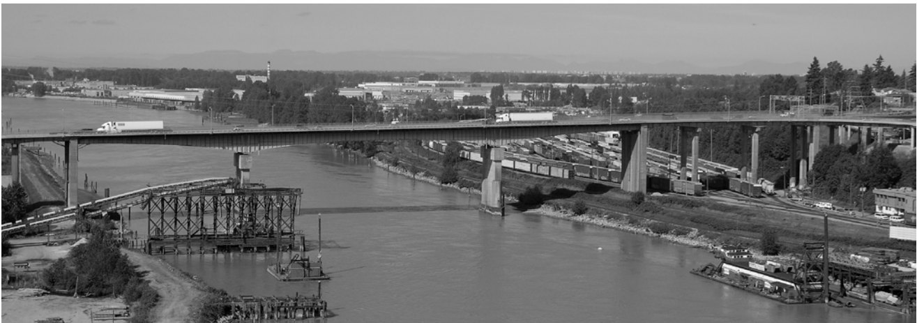
QUEENSBOROUGH HIGHWAY BRIDGE (2007)
