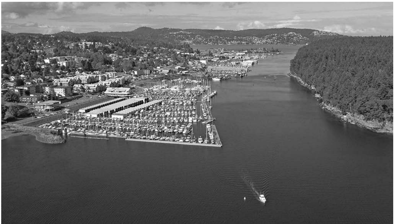
NEWCASTLE ISLAND PASSAGE LOOKING NW (2005)
