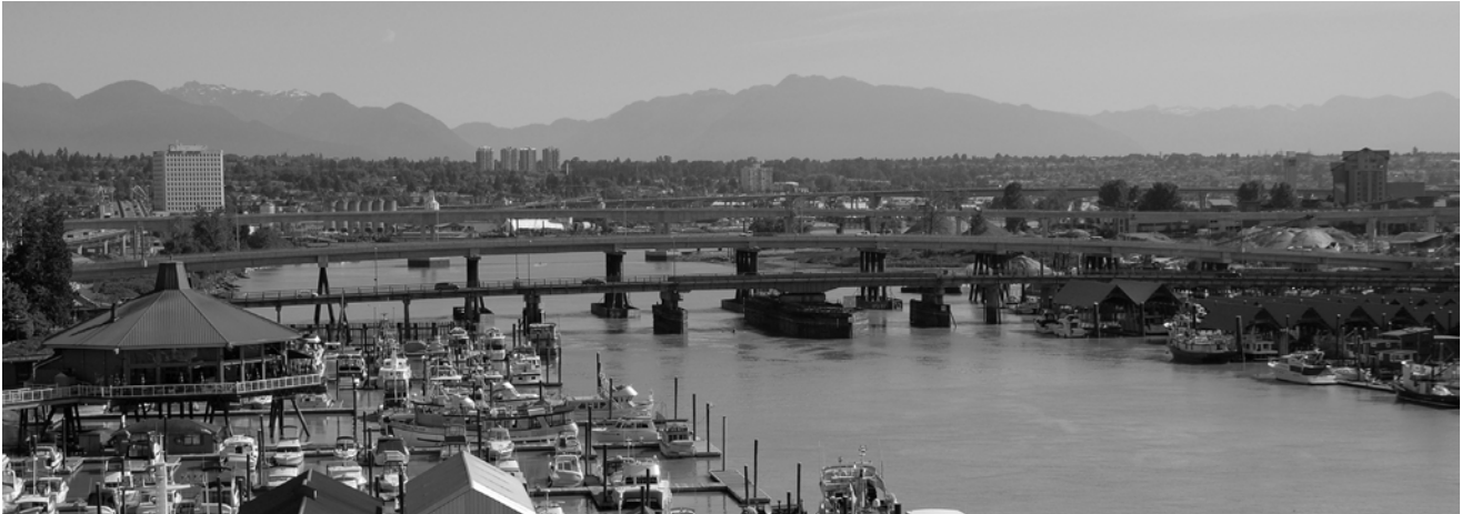
MIDDLE ARM SWING BRIDGE (2007)
