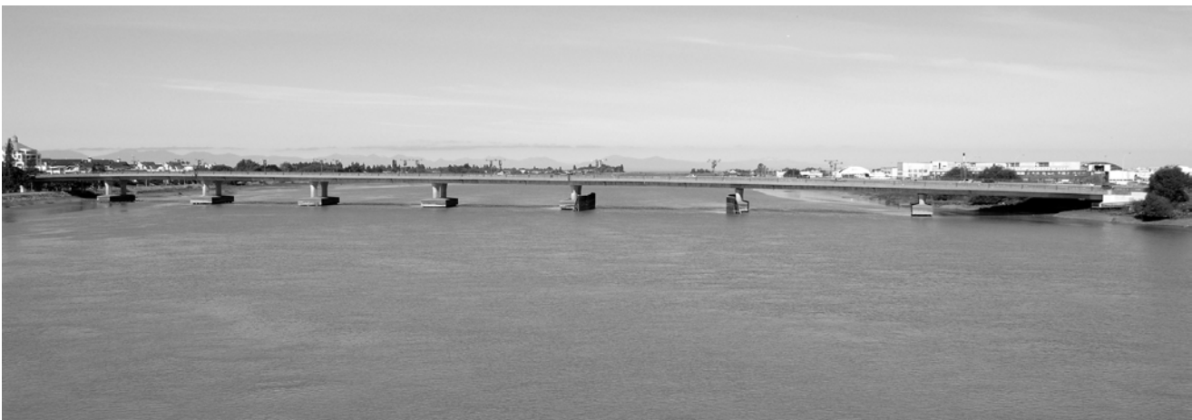
NO. 2 ROAD BRIDGE (2007)
