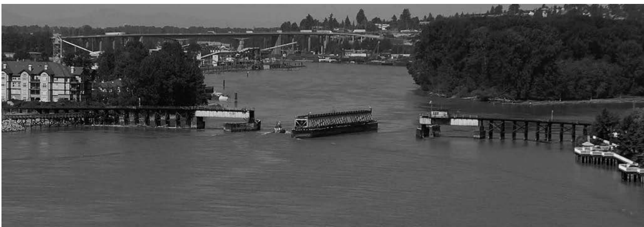
QUEENSBOROUGH RAILWAY BRIDGE (2007)
