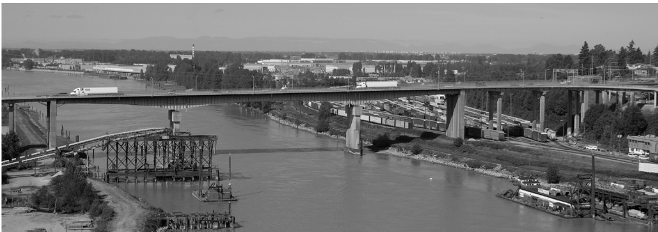
QUEENSBOROUGH HIGHWAY BRIDGE (2007)
