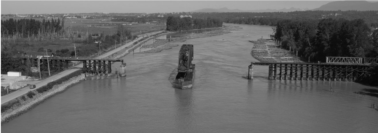
CANADIAN NATIONAL RAILWAY BRIDGE (2007)
