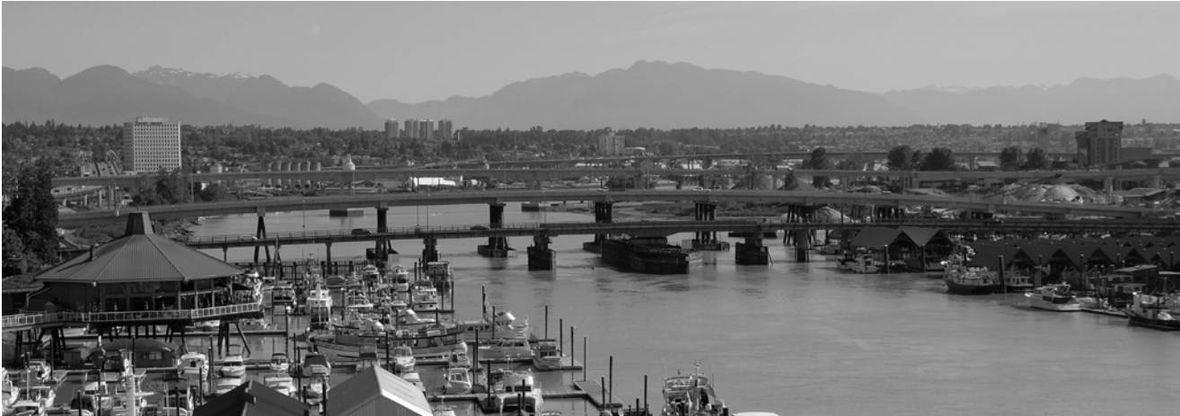
MIDDLE ARM SWING BRIDGE (2007)
